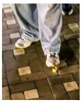
Figure 38: Conduit protruding above the sidewalk level.
