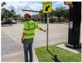
Figure 32: Inaccessible pushbutton location.
