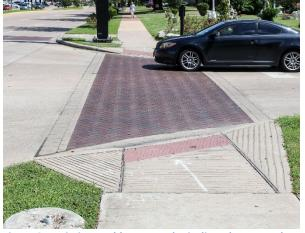
Figure 31: Missing pushbutton and misaligned truncated domes.
