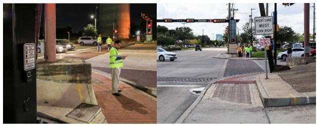
Figure 41: Pushbutton away from beginning of crosswalk.
