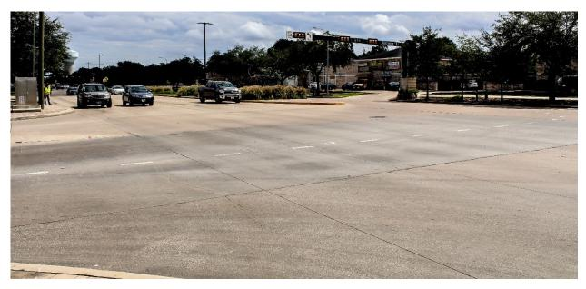
Figure 36: Dotted line extension markings ("cat tracks") through intersection aligned to outside lanes of Bellaire.
