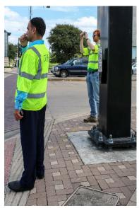
Figure 44: Pushbutton not located next to level landing.
