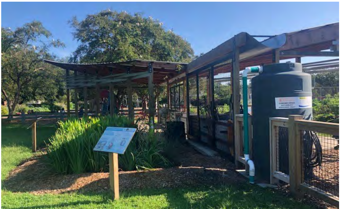
Corine Jones Community Garden with rain garden and rainwater harvesting system installed by the Master Rain Gardener course through Clemson Cooperative Extension Image credit: Charleston Rainproof
