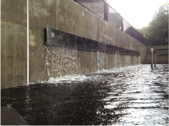
Waterwall on the Bentheplein designed by the Urbanisten, Image credit: Jurgen Bals
