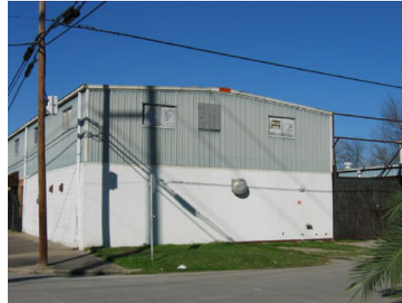
Example: A non-contributing structure.
