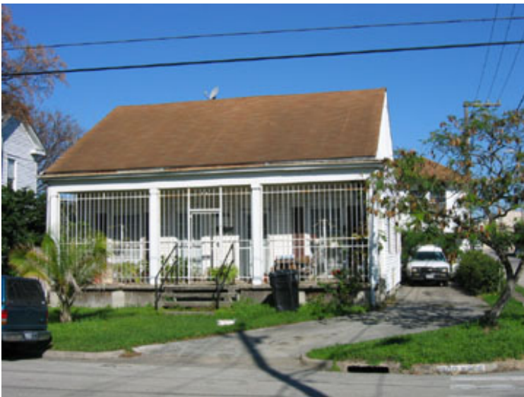
The residence at 1904 Kane is a potentially contributing structure.
