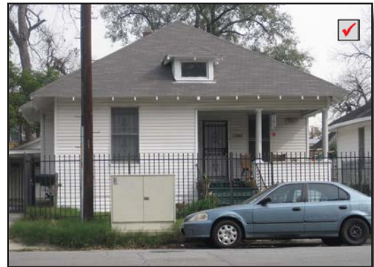
Typical hipped roof with dormer
