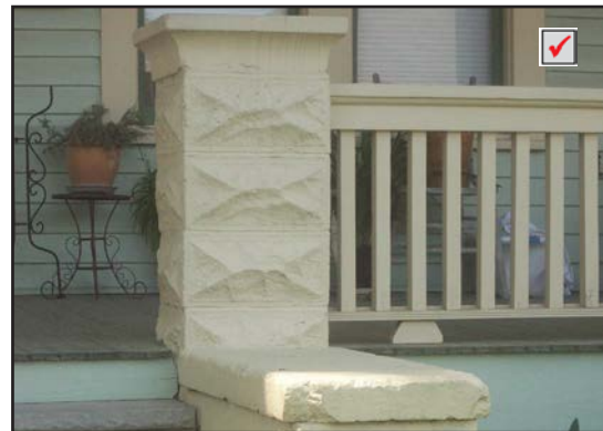
Cast concrete block porch column/base
