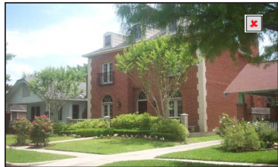
Incompatible infill (size, style) between historic houses
