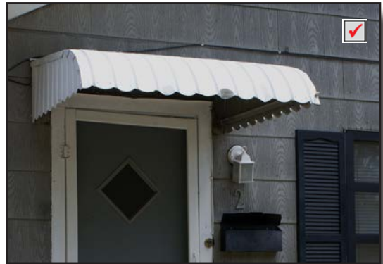
Modest awning over front door
