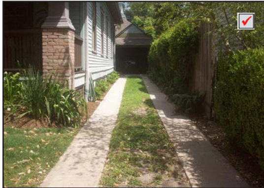
Poured concrete driveway (strips)
