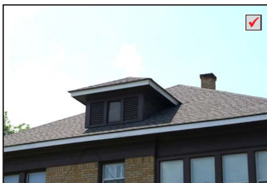
Original dormer with window and vents
