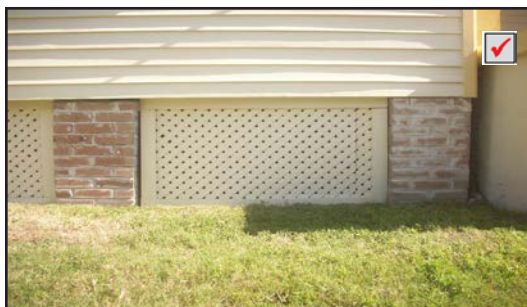
Lattice panel, framed between piers
