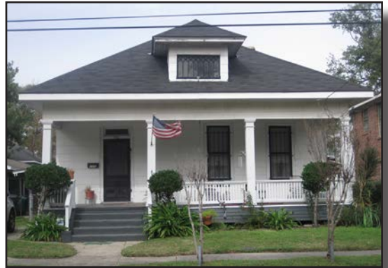
Hipped roof with full-width porch
