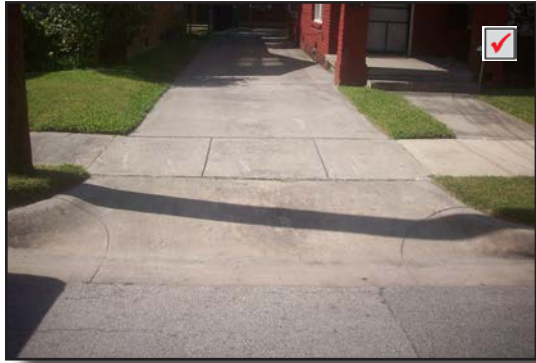
Poured concrete driveway
