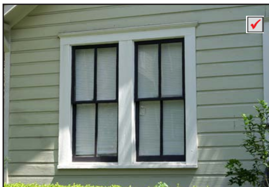
Two-over-two window, typical in Queen Anne houses
