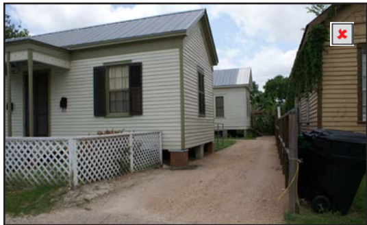
Gravel driveway — not recommended
