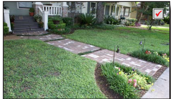
Walkway constructed of brick pavers
