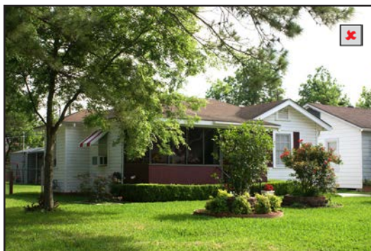
Incompatible screened-in porch
