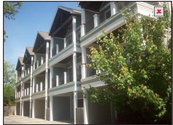
Streetscape in neighborhood of high density townhouses
