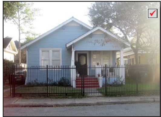
Typical gabled roof
