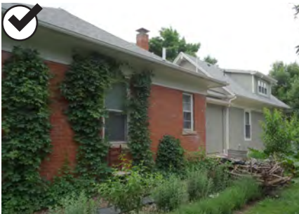
This is a compatible rear addition even though it is slightly taller than the historic building. It is compatible because it is offset, separated by a hyphen and uses compatible materials.
