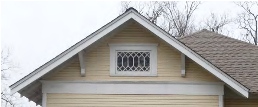
Maintain traditional overhangs; these contribute to the perception of the building's historic scale and its character.
