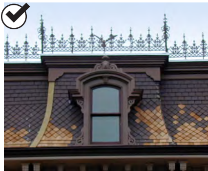
Patch and replace damaged areas of the existing roof.
