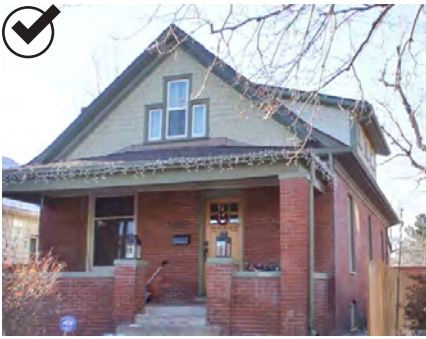
Locate a new single dormer in a location that is toward the rear of the house and on the side of the roof that is as close to the middle of the lot as possible.
