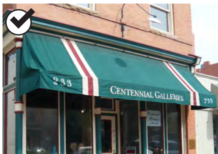
Maintain awning frames and any moving parts.
