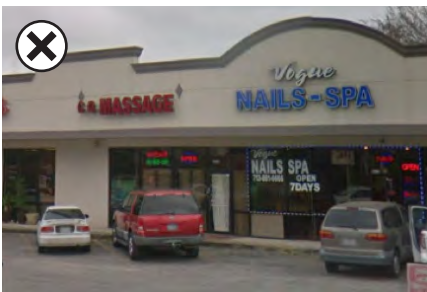
A noncontributing strip center with internally lit plastic channel letter signs
