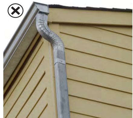
Do not cut back a roof eave so it is flush with the wall.
