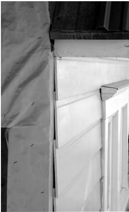
Installation of fiber-cement siding
