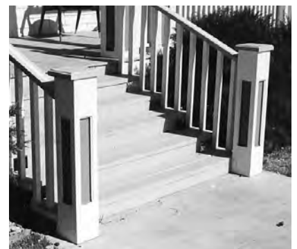
After: Handrail repaired and the post replaced in kind.
