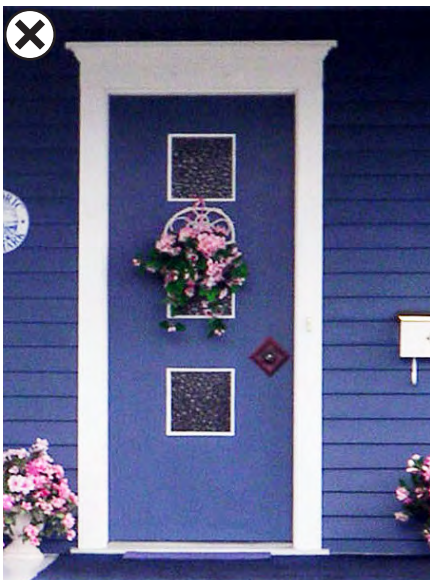
This replacement door is a style popular in the mid-20th century and would be inappropriate for a contributing building in the Houston Heights Historic Districts.
