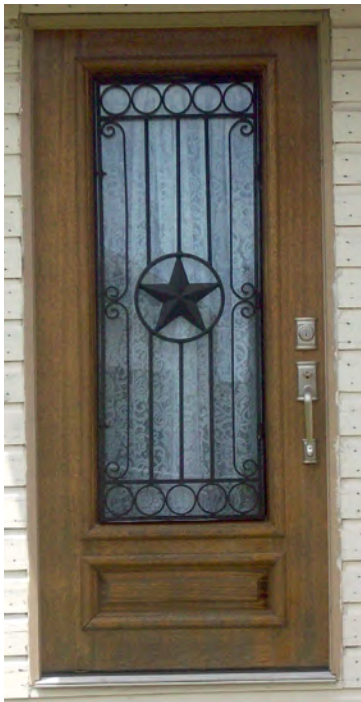
This replacement door with ornate, faux "leaded" glass would be inappropriate on most historic buildings.
