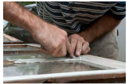
Replacing glazing putty © iStockPhoto.com/Elaine Odell
