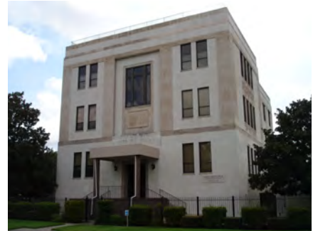
1918 Masonic Lodge Building
