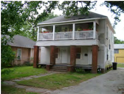
Wilkins House, 1541 Ashland Street
