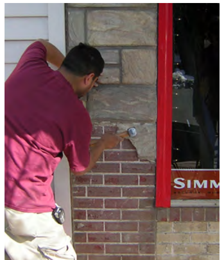
Restoration to a previous period by removal of "stone" paneling
