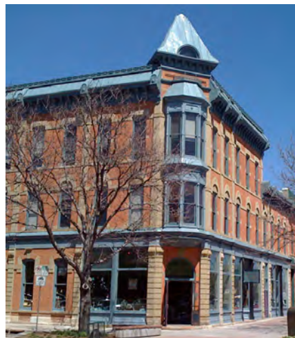
The same building after rehabilitation
