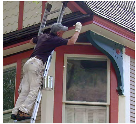
Preservation of historic materials
