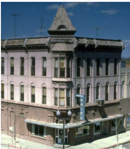
A commercial building before rehabilitation
