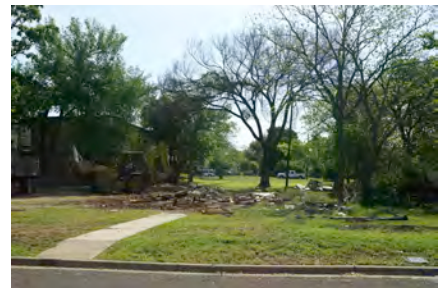
Examples of demolition
