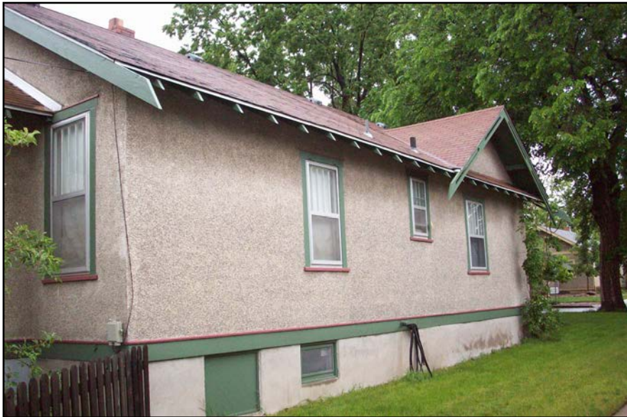
Rear part of left side wall
