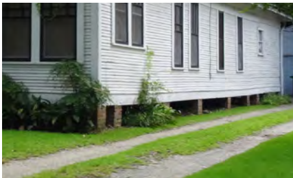
Maintain paved and unpaved driveways beside the house.
