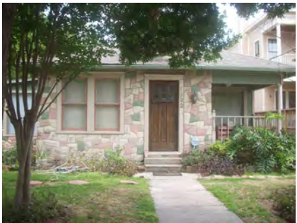
Faux stone panelized wall cladding (not appropriate for the Houston Heights Historic Districts)
