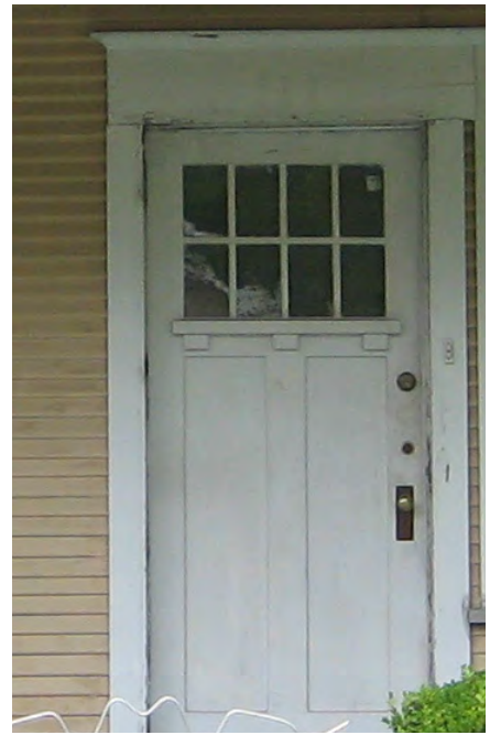
Preserve the proportions of a historic door and its opening.
