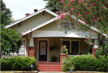
A front gabled roof
