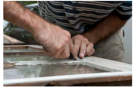
Replacing glazing putty © iStockPhoto.com/Elaine Odell
