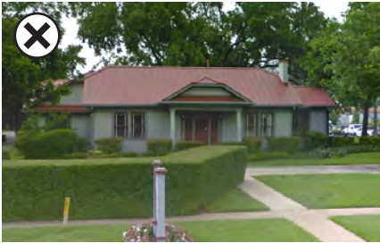
The red metal roof on this house is more appropriate for a commercial building, not a residential one.
