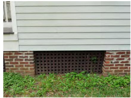
A foundation with masonry piers
