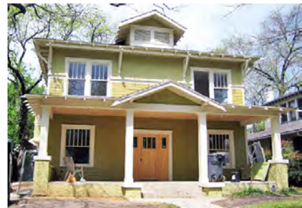
Reconstruction of the porch on a historic house: (top) before; (bottom) after
