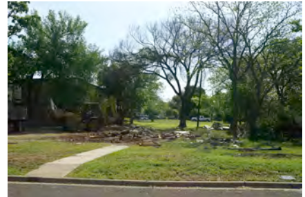
Examples of demolition
