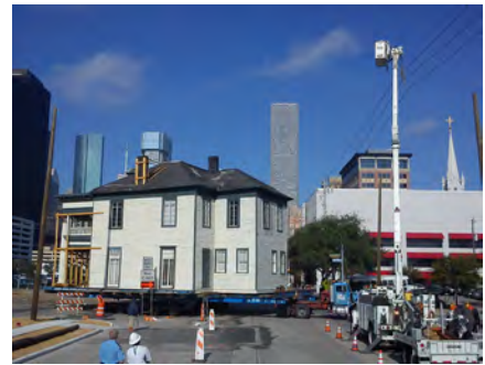
These houses were relocated from various locations within the City of Houston.
