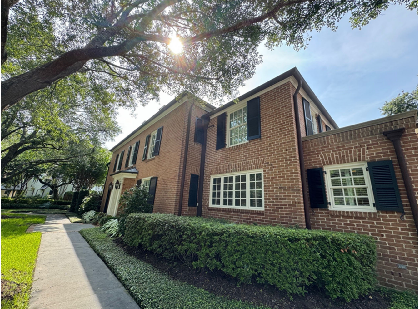
Photo 6: Oblique view of the north (front) elevation of the Dr. and Mrs. Robert A. Johnston House. Camera facing southeast. Photo by HOP staff Cara Quigley, July 2024.
