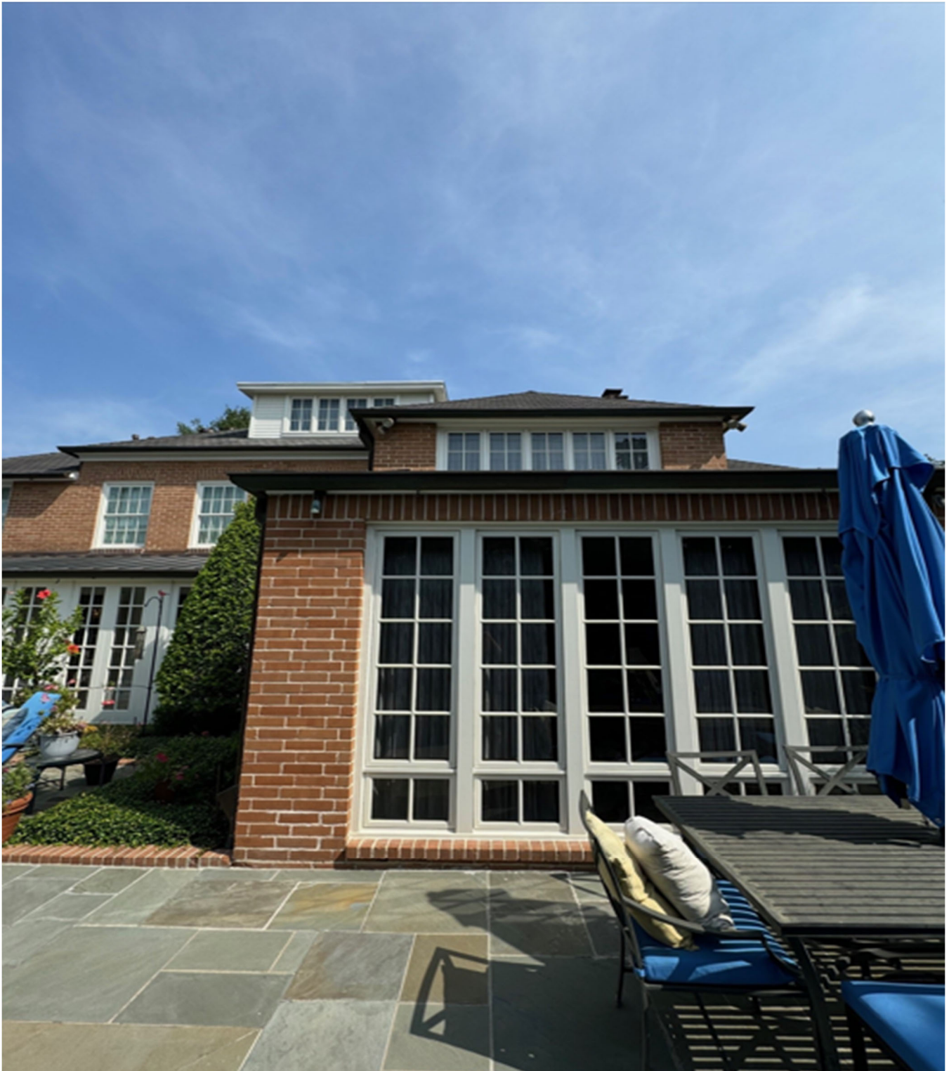
Photo 11: South (rear) elevation of the Dr. and Mrs. Robert A. Johnston House. Camera facing north. Photo by HOP staff Cara Quigley, July 2024.
