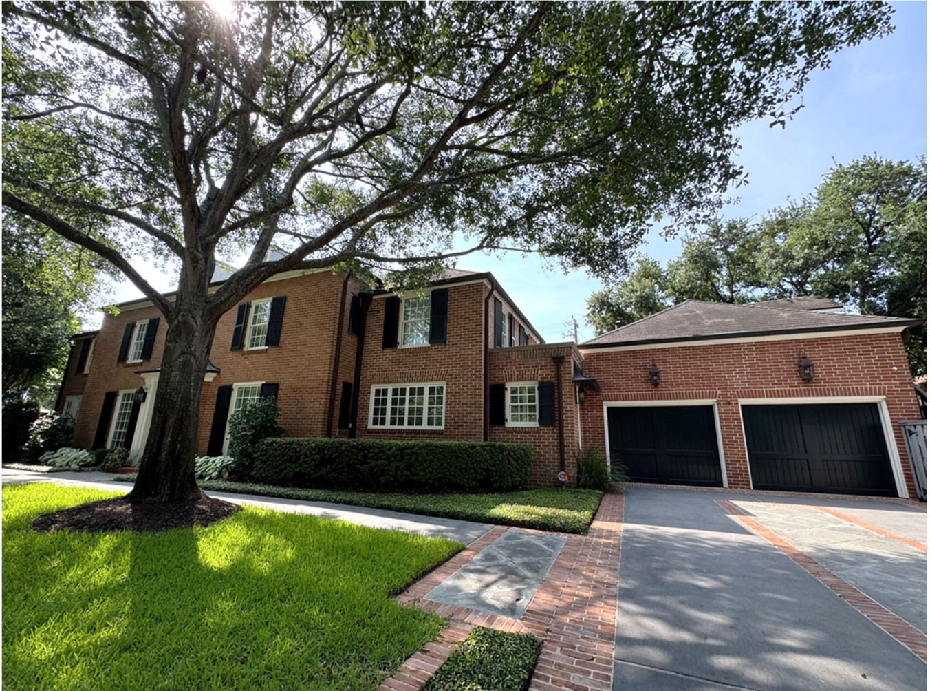
Photo 5: Oblique view of the north (front) elevation of the Dr. and Mrs. Robert A. Johnston House and garage. Camera facing southeast. Photo by HOP staff Cara Quigley, July 2024.
