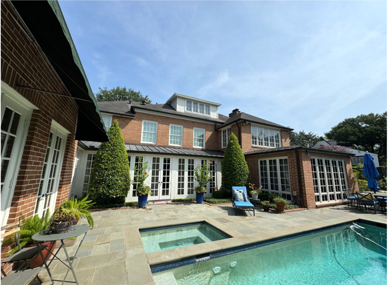
Photo 13: Oblique view of the south (rear) elevation of the Dr. and Mrs. Robert A. Johnston House. Camera facing northeast. Photo by HOP staff Cara Quigley, July 2024.
