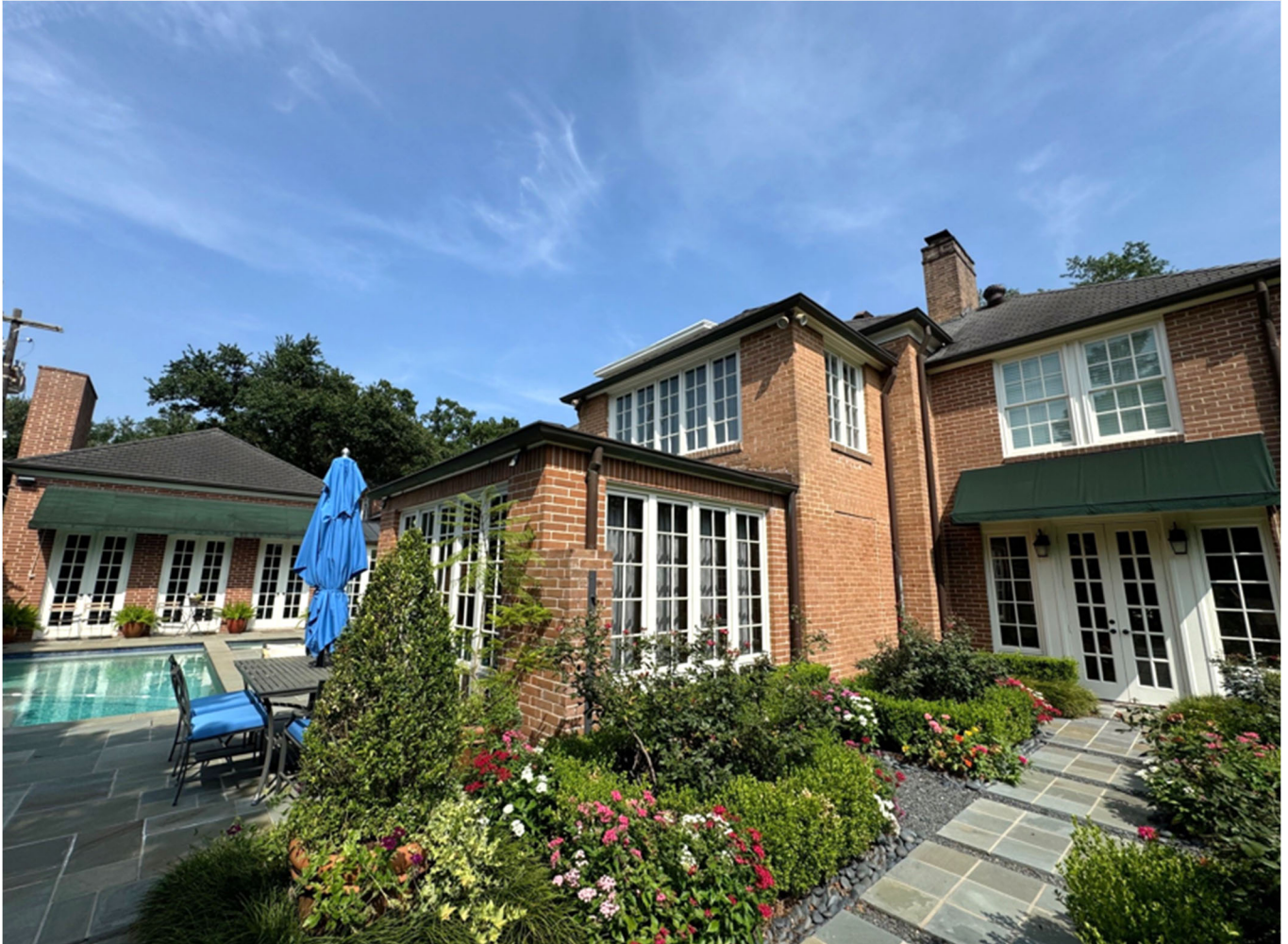
Photo 10: Oblique view of the south (rear) elevation of the Dr. and Mrs. Robert A. Johnston House. Camera facing northwest. Photo by HOP staff Cara Quigley, July 2024.
