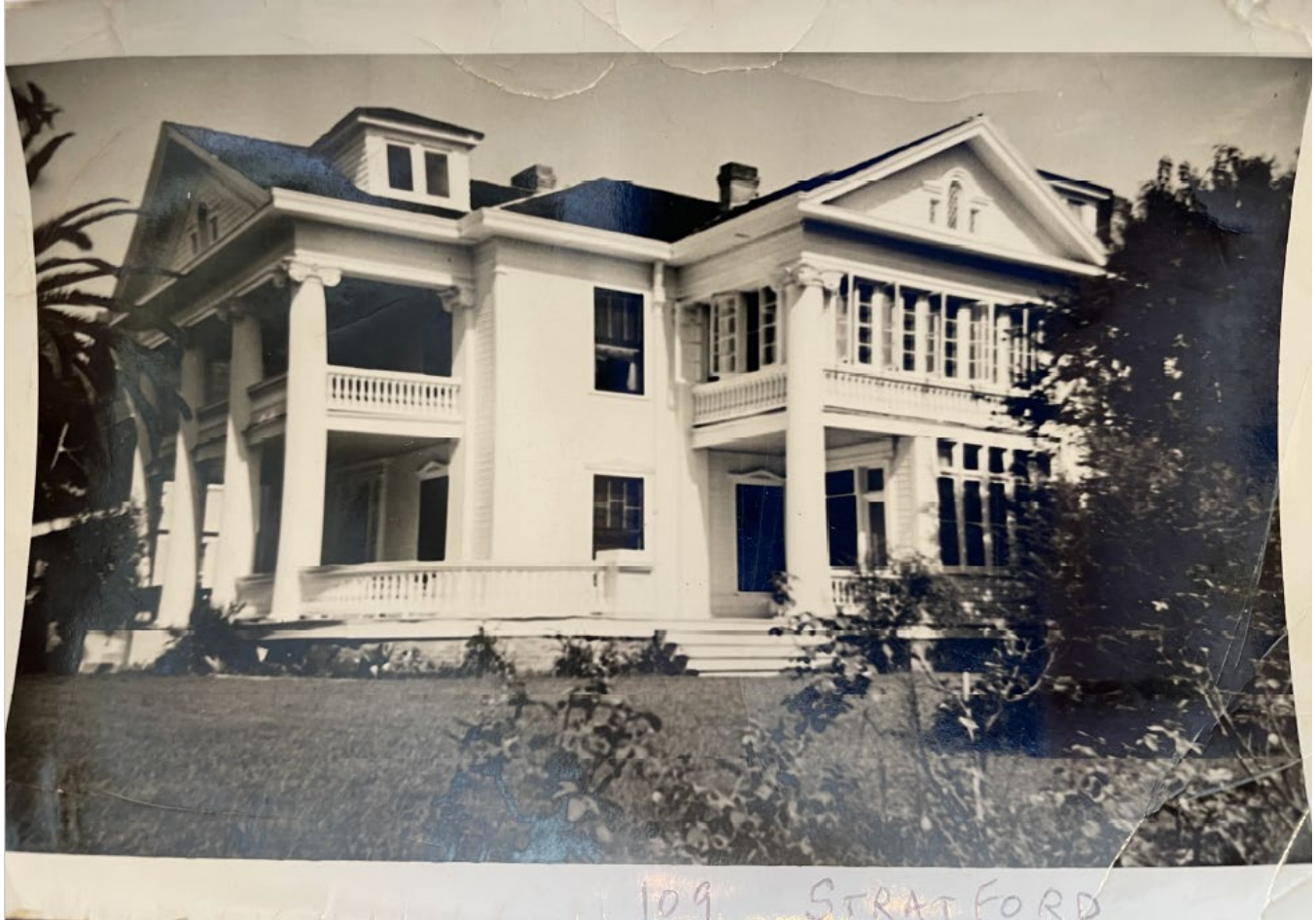
Figure 3: Historic photograph of the John S. Stewart House c.1924-1926. The photo shows a circular wrap-around porch previously connected the south (front) portion of the house to the side wing projecting from the east (right) elevation. Camera facing northwest. Photo courtesy of applicant, 2024.
