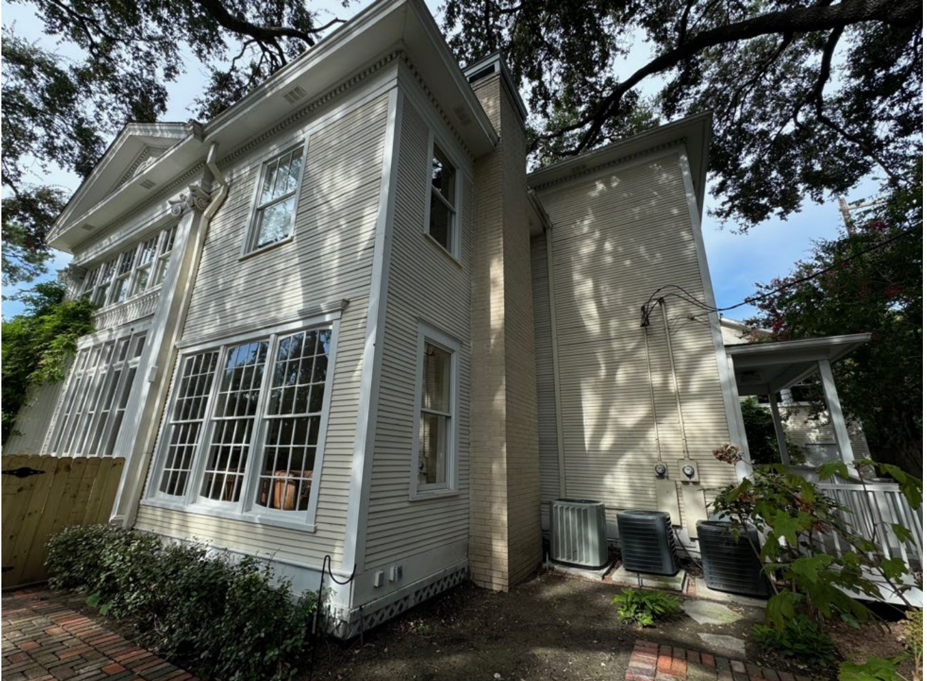
Photo 9: Oblique view of the northeast (right/rear) elevation corner of the John S. Stewart House. Camera facing southwest. Photo by HOP staff Cara Quigley, August 2024.
