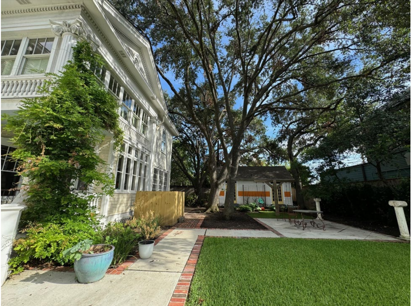
Photo 4: Oblique view of the east (right) elevation and lawn looking to the rear of the lot with noncontributing accessory structure (not included in Protected Landmark designation) of the John S. Stewart House. Camera facing north. Photo by HOP staff Cara Quigley, August 2024.
