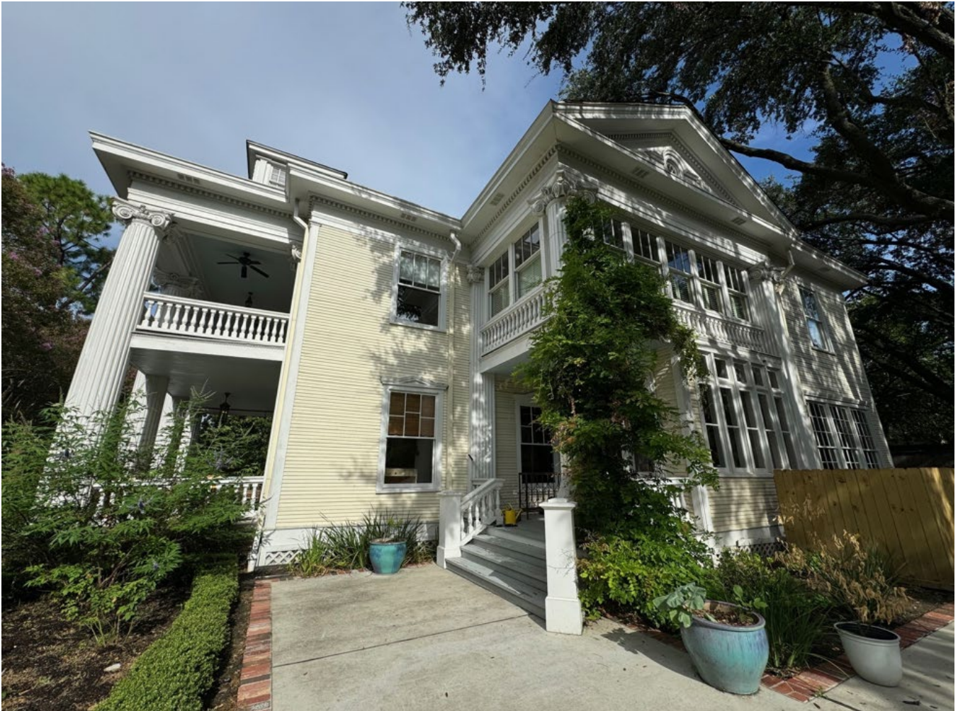
Photo 5: Oblique view of the east (right) elevation and projecting side wing of the John S. Stewart House. Camera facing northwest. Photo by HOP staff Cara Quigley, August 2024.
