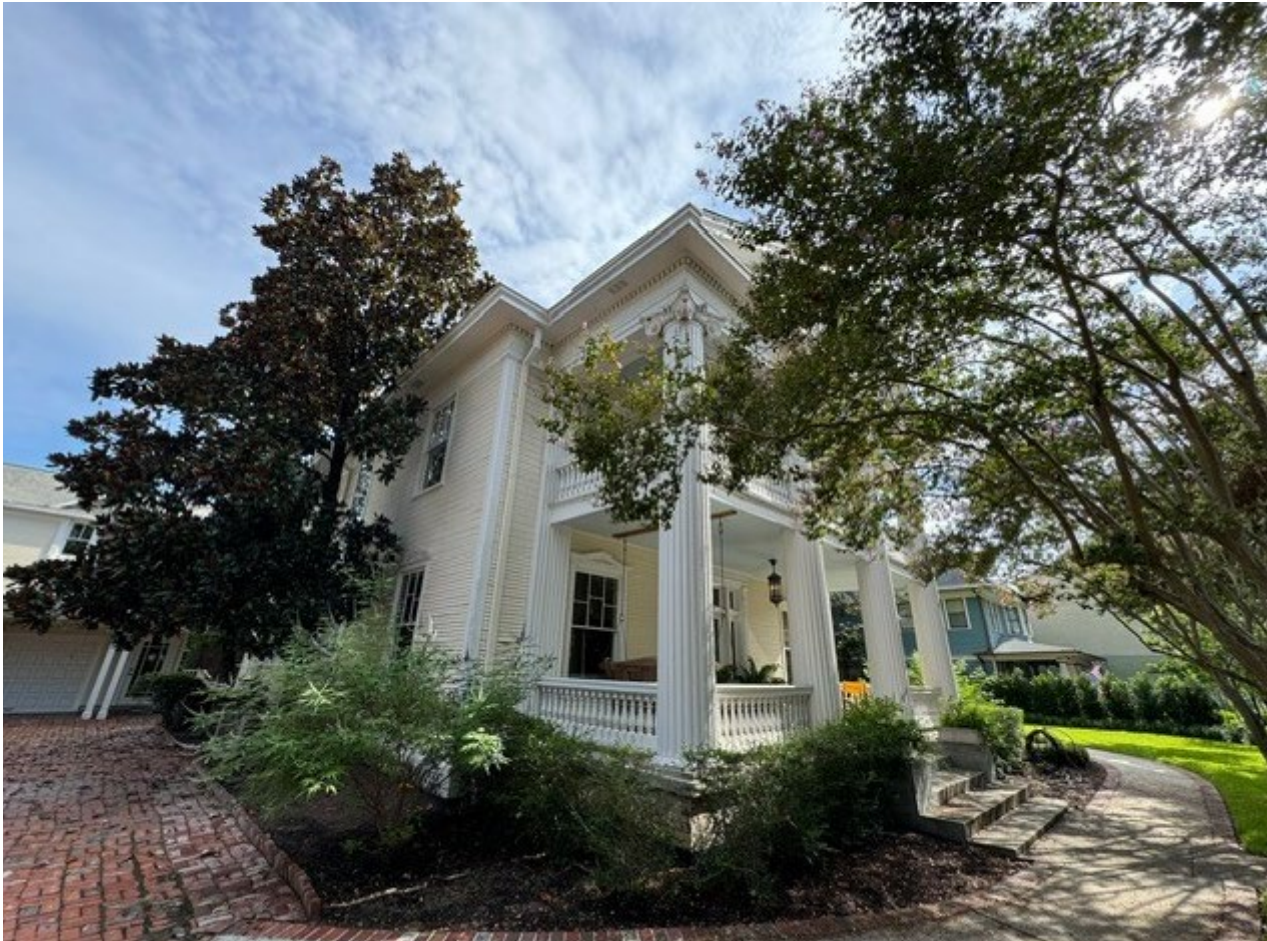
Photo 15: Oblique view of the southwest (front/left) elevation corner of the John S. Stewart House. Camera facing northeast. Photo by HOP staff Cara Quigley, August 2024.
