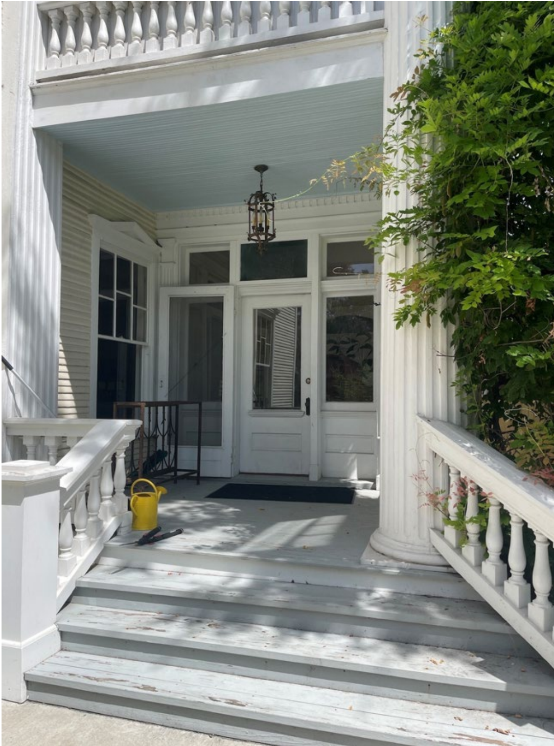
Photo 3: Side wing covered porch projecting off of the east (right) elevation of the John S. Stewart House. Camera facing north. Photo by applicant, August 2024.
