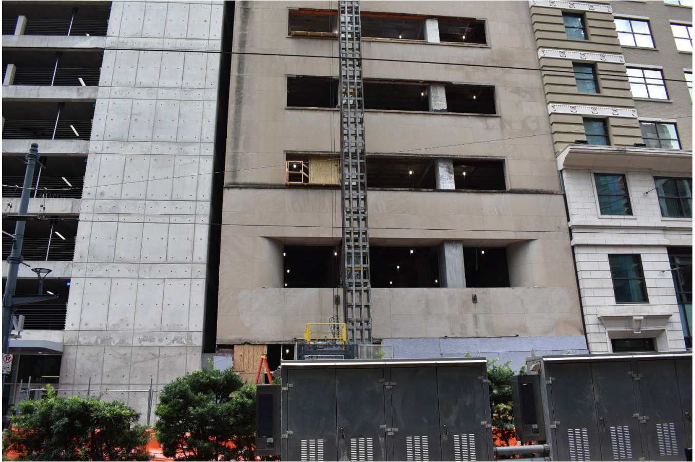
Photo 4: East (front) elevation facing Main Street. Detail view of inset second floor balcony. Camera facing northwest. Photo by applicant, 2024.
