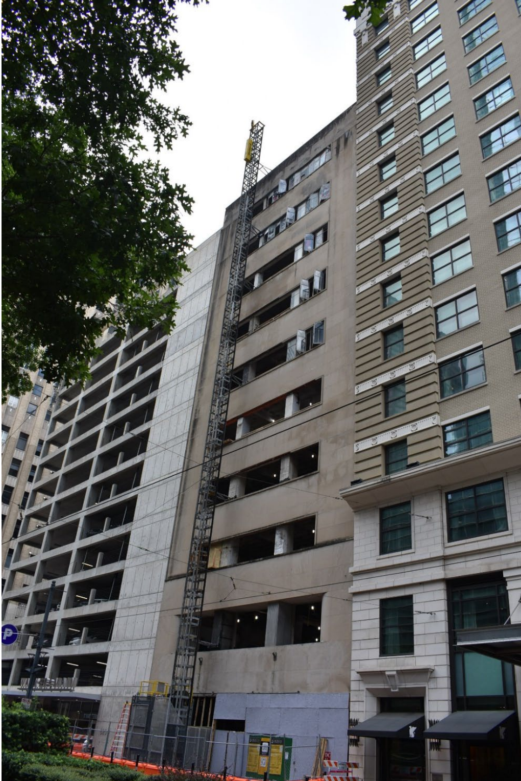
Photo 2: Oblique view of the east (front) elevation facing Main Street. Camera facing west. Photo by applicant, 2024.
