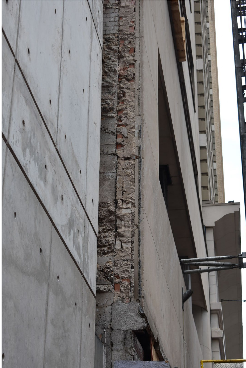
Photo 7: East (front) elevation facing Main Street. Detail view of exterior limestone and brick façade. Three-quarter view, camera facing north. Photo by applicant, 2024.
