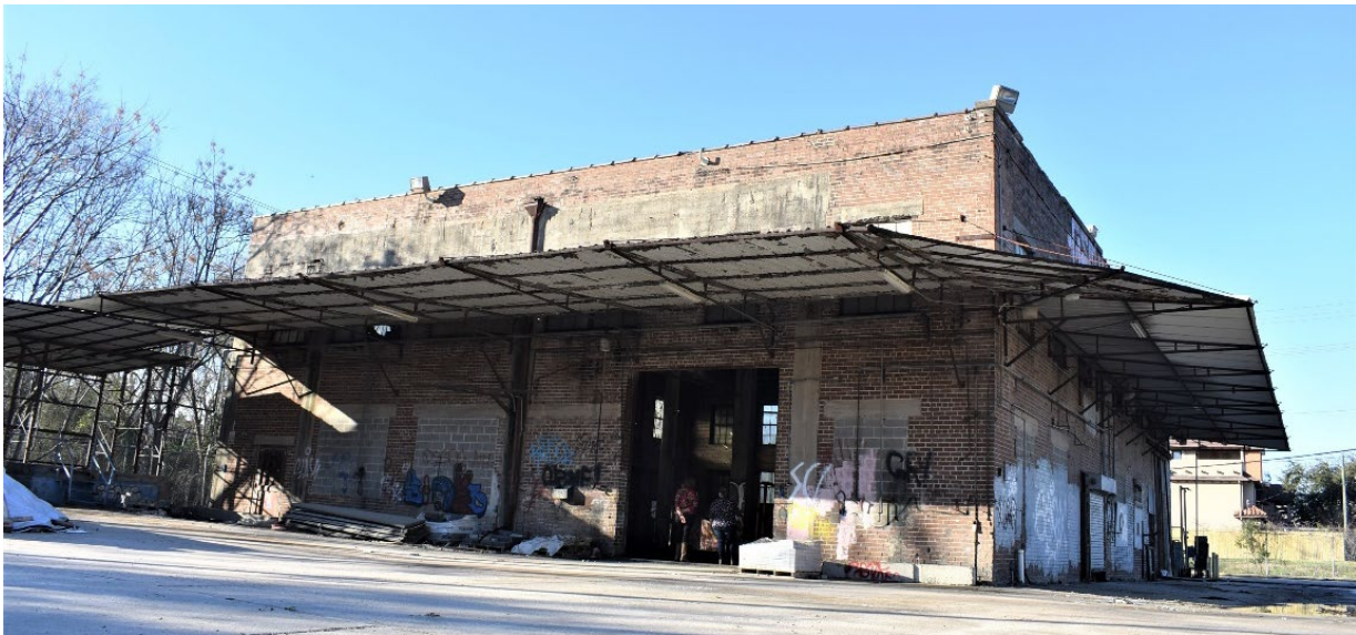
Photo 28 Boiler and Engine House; South elevation; view north
