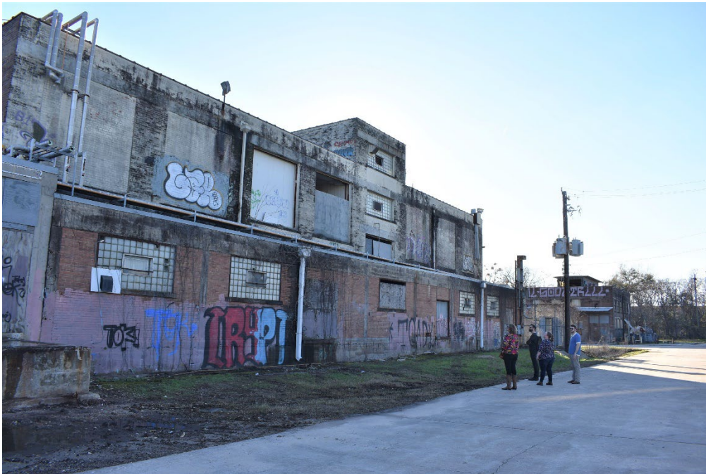
Photo 4 Swift & Co. Packing Plant; North elevation; view southwest
