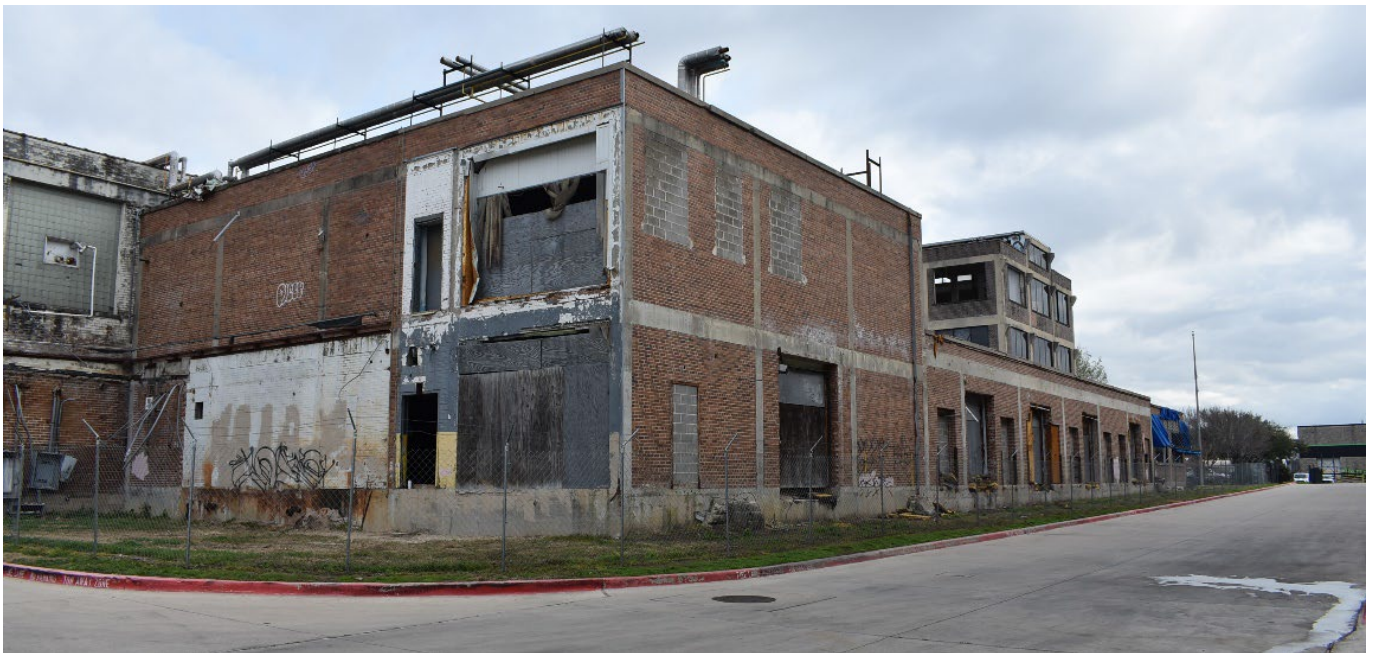
Photo 6 Swift & Co. Packing Plant; Southwest corner; view northeast
