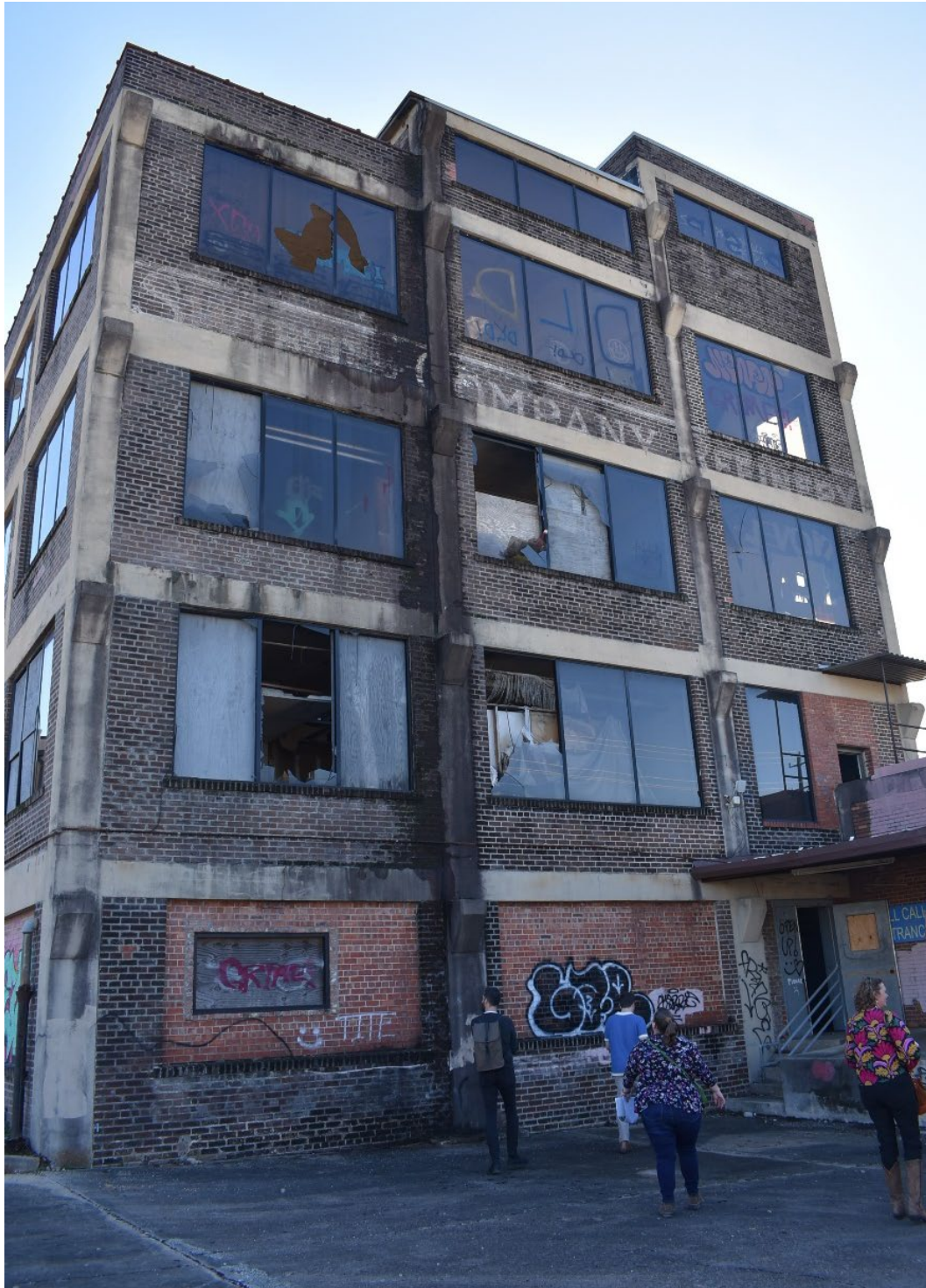
Photo 2 Swift & Co. Packing Plant; North elevation; view south
