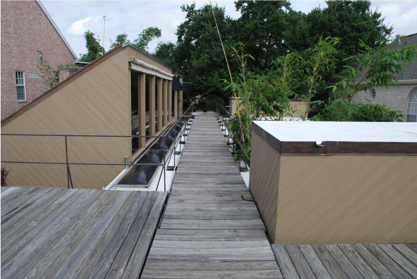
ROOF DECK – LOOKING TOWARDS STREET
