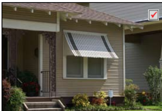
Metal awning over window
