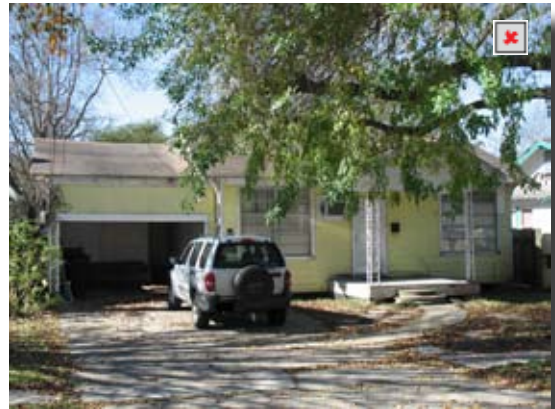
Attached garage, attached to side of house in front half of property
