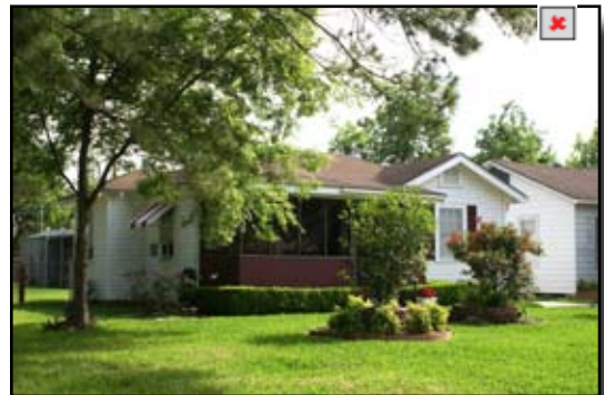
Incompatible screened-in porch
