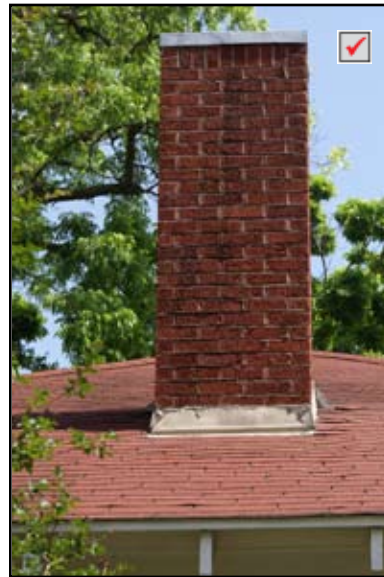
Chimney located on an interior wall
