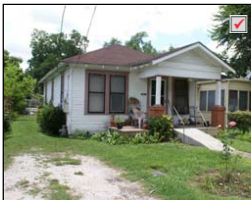
Concrete ramp to front porch, with handrails
