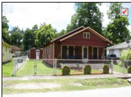
Typical gabled roof
