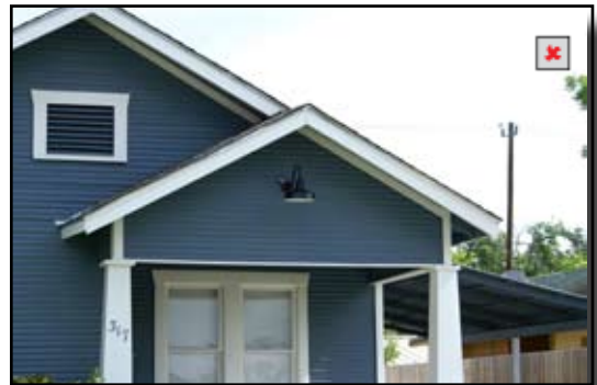
Utility light placed on front of house — not recommended
