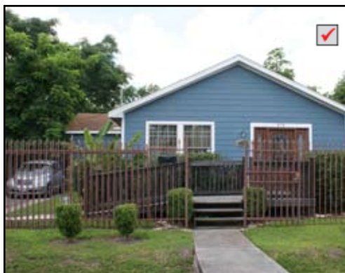
Wooden ramp to front deck
