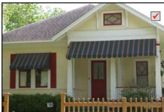
Fabric awning over window (compatible) and porch (incompatible)
