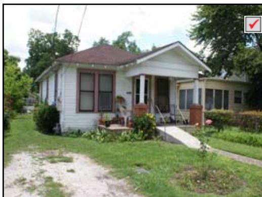
Typical hipped roof with front gable
