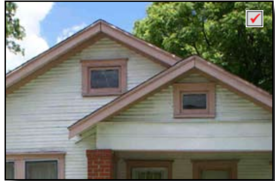
Original windows in gables
