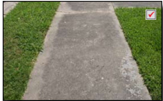
Poured concrete sidewalk
