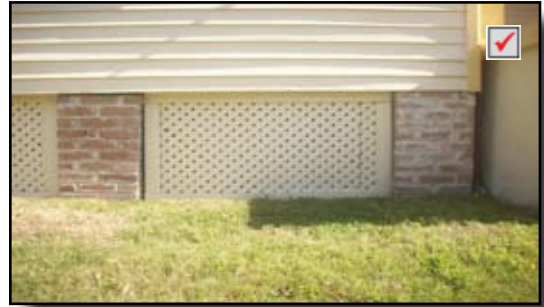
Lattice panel, framed between piers
