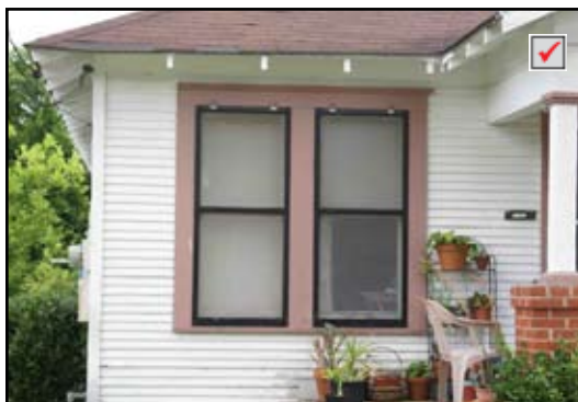
One-over-one original window with exterior storm windows
