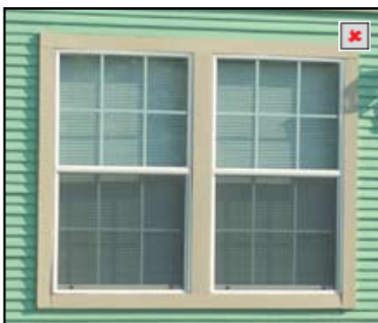
Six-over-six window (not original) with interior muntins
