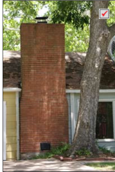
Chimney located on an exterior wall
