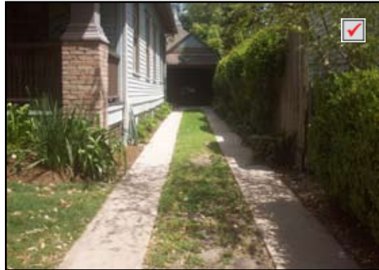
Poured concrete driveway strips
