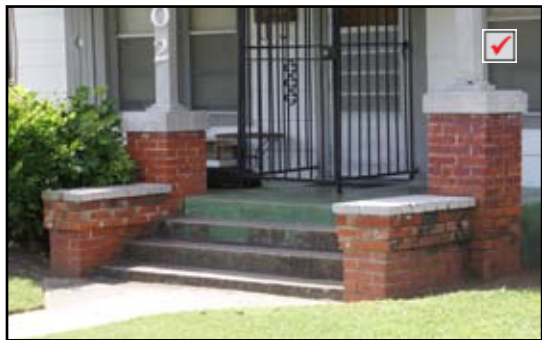
Brick porch column/base
