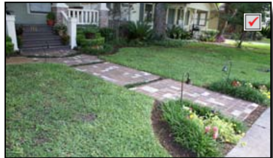
Walkway constructed of brick pavers
