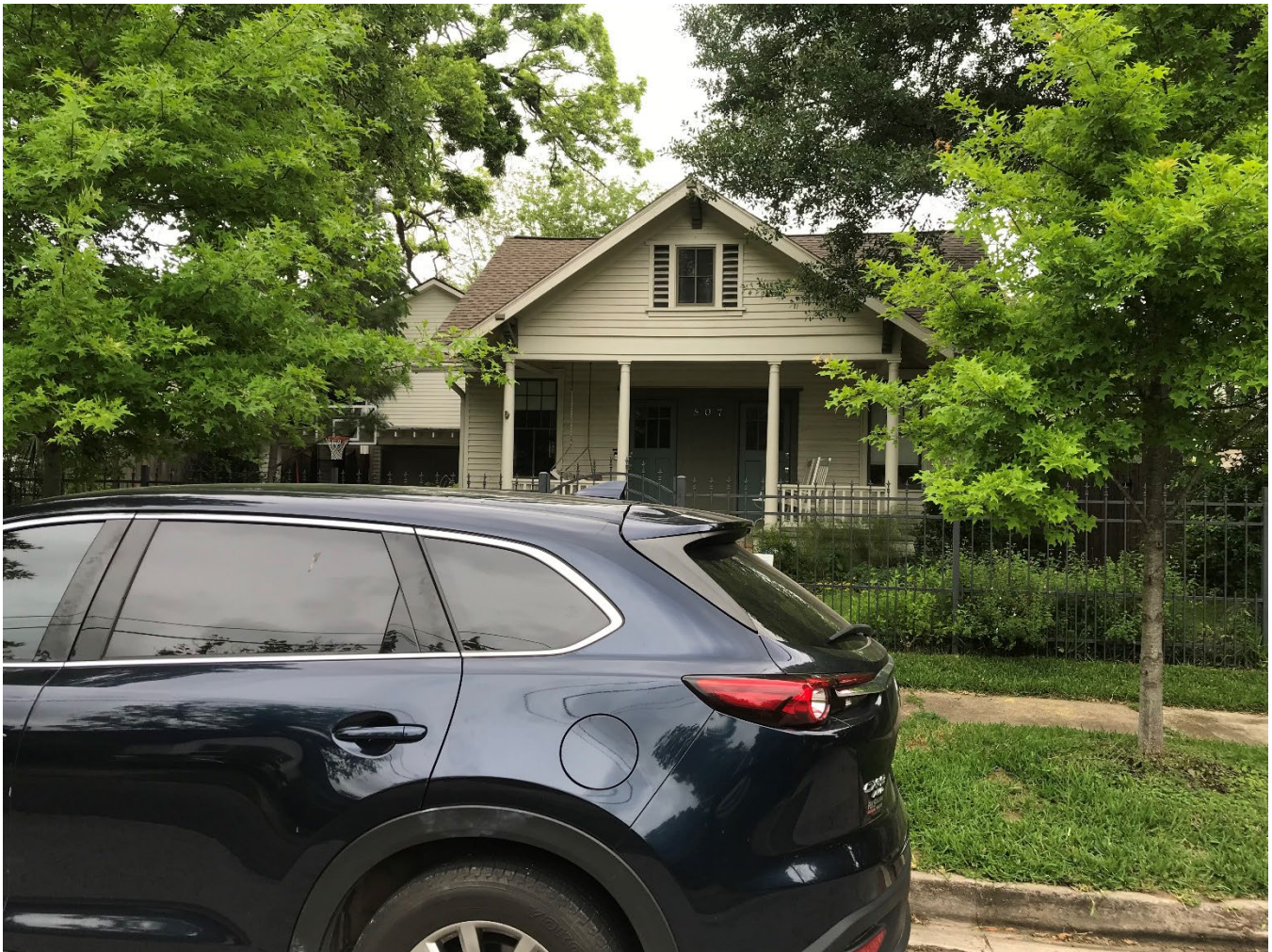
Figure 4 - Before 2nd Story Added
