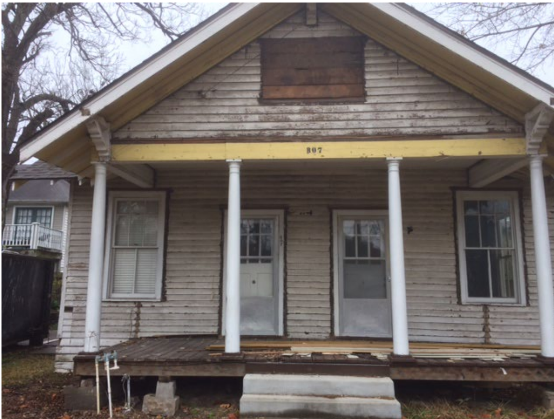
Figure 1 - 2018 After Synthetic Siding Removed
