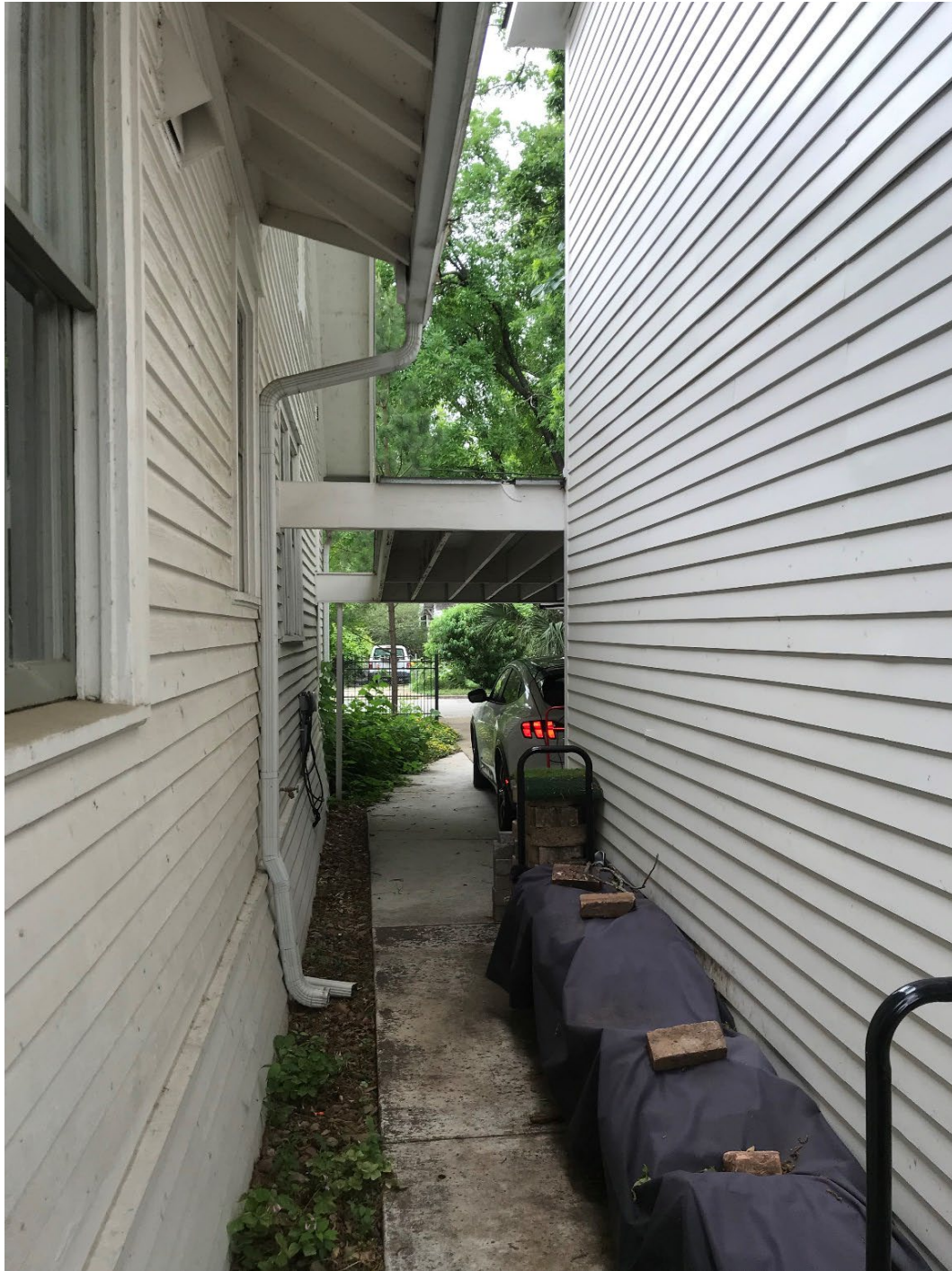
Figure 9 - View Looking Between House and Garage Toward Front
