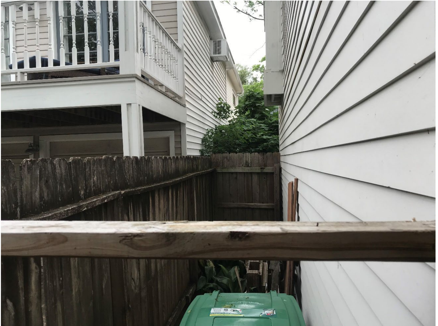
Figure 8 - View Looking Towards Rear at Property Line
