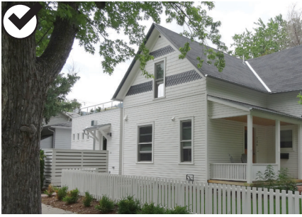
This rear addition is compatible. It is set behind the primary contributing buildings, is separated by an inset, and is subordinate in height, mass and scale. It is also a successful contemporary addition.
