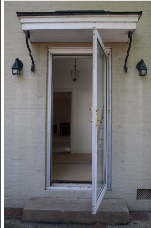
11. Non-original side door (likely added during 1977 remodel) at SW corner of W elevation of main house (along Woodhead Street) in place of an original window. View W.
