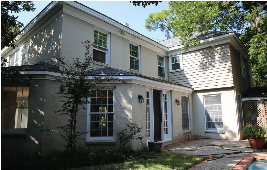
Exhibit 6: September 2022 photo of rear, N elevation of main house. View SE. Two-story addition and one-story carport (along Woodhead Street) from 1977 remodel on right. First-floor, angled addition along rear, N elevation added during a 1988 remodel. Second-floor extension also added to the rear, N elevation during 1988 remodel. Bay window along E elevation (left) also added during 1988 remodel.
