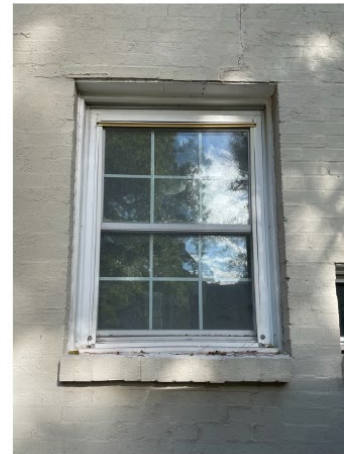
D2 - EXISTING: Non-original window on west elevation facing Woodhead Street. Added during 1977 renovation of kitchen.
