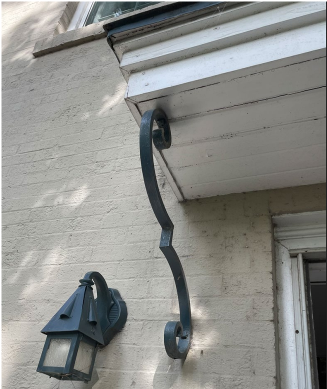
Top of existing side door entryway, may have been window
