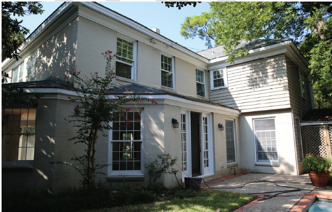
Exhibit 6: September 2022 photo of rear, N elevation of main house. View SE. Two-story addition and one-story carport (along Woodhead Street) from 1977 remodel on right. First-floor, angled addition along rear, N elevation added during a 1988 remodel. Second-floor extension also added to the rear, N elevation during 1988 remodel. Bay window along E elevation (left) also added during 1988 remodel.
