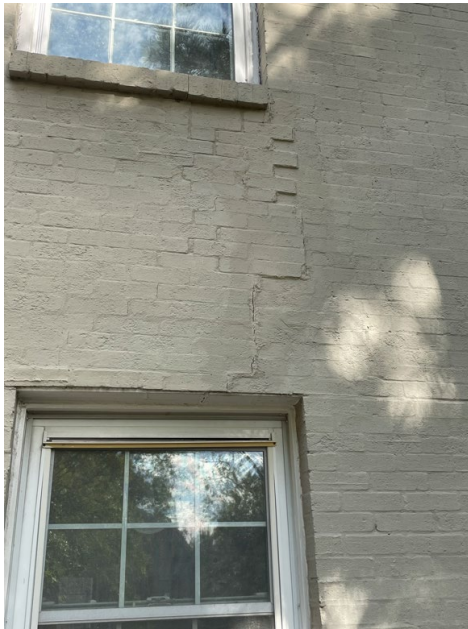
Current damage located near c. 1970 addition
