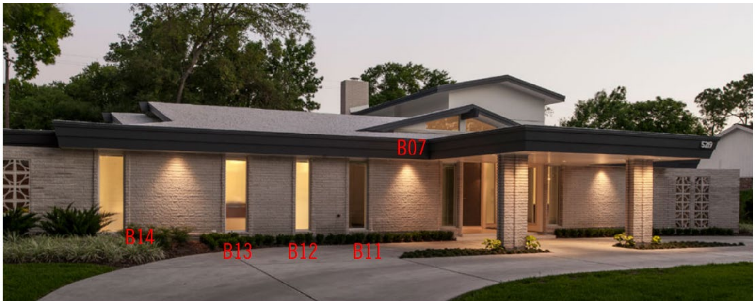
01 - Front (north) elevation, showing windows B14~B11, and B07
