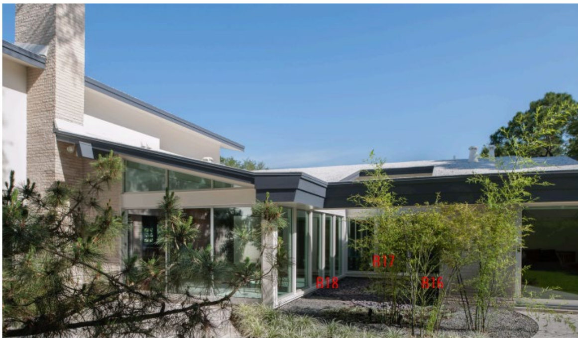
12: Back (south) elevation, locations of windows B16-B18 in rear courtyard.
