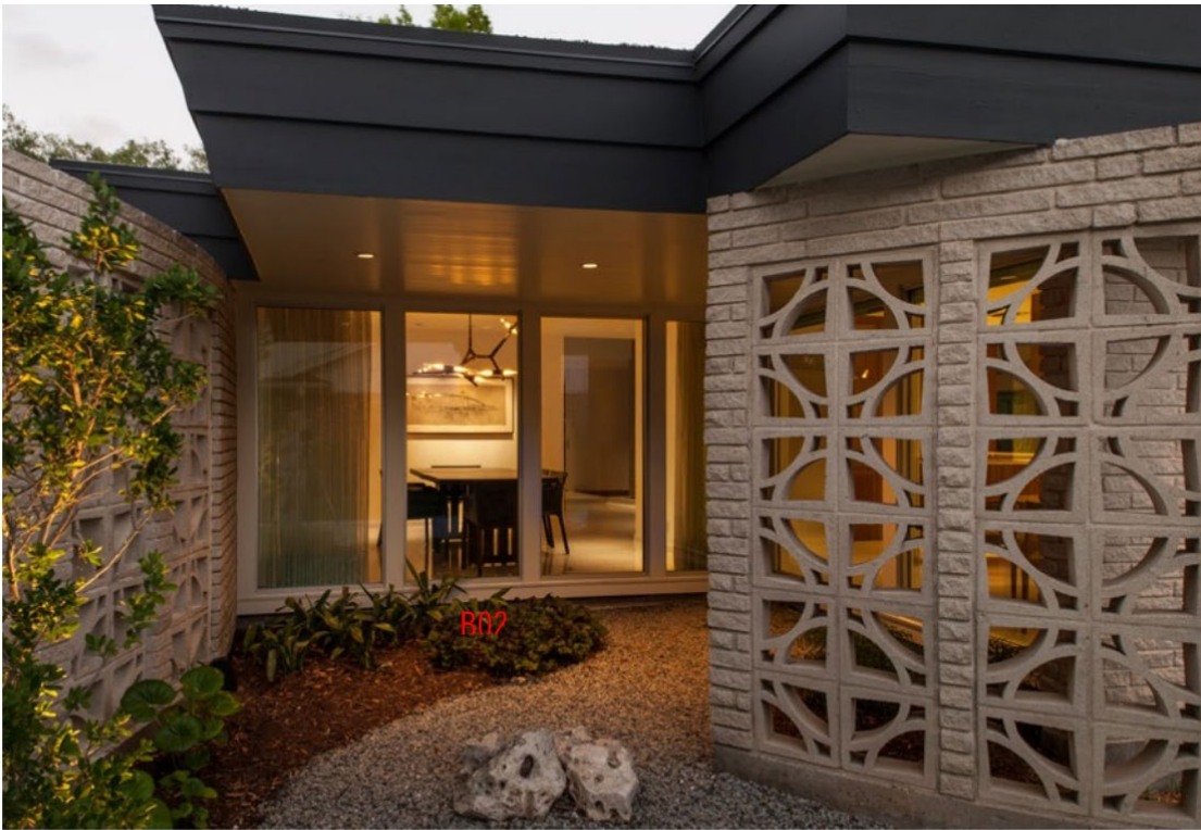
04 – West (side) partial elevation at front of house, showing window unit B02
