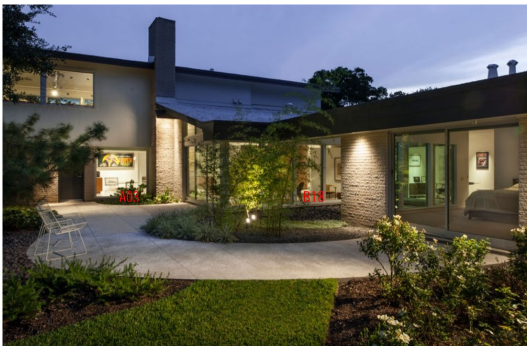
07 – South (rear) elevation at original house and East (side) elevation at rear addition, showing windows A03 and B18
