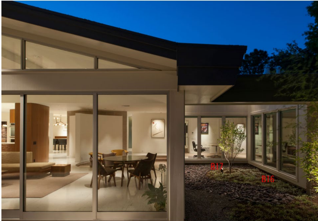
08 – South (rear) partial elevation, showing windows B16 and B17
