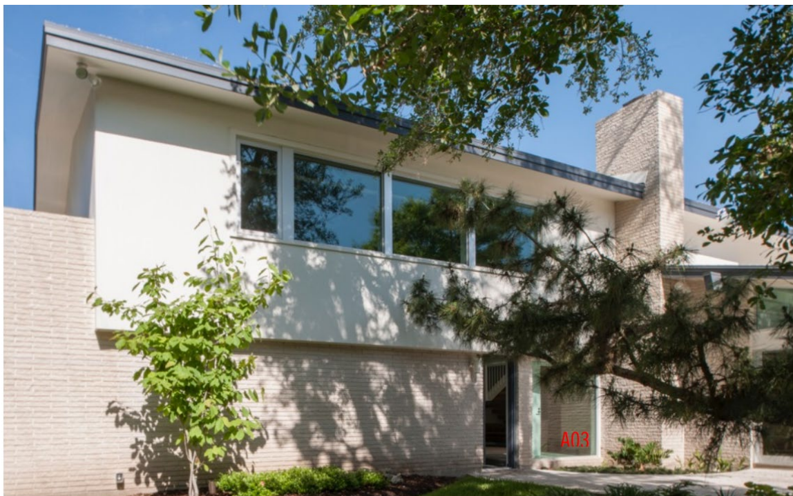
06 – South (rear) elevation at addition, showing window A03
