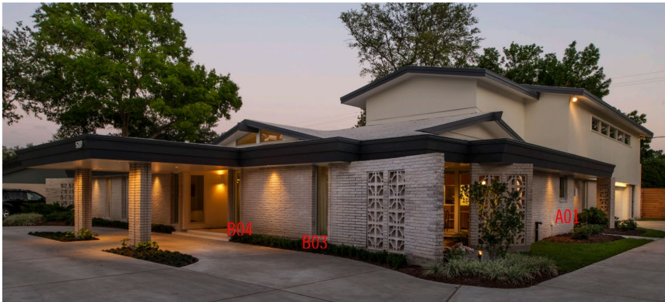
03 – Front (north) and West (side) elevations, showing windows A01, B03 and B04
