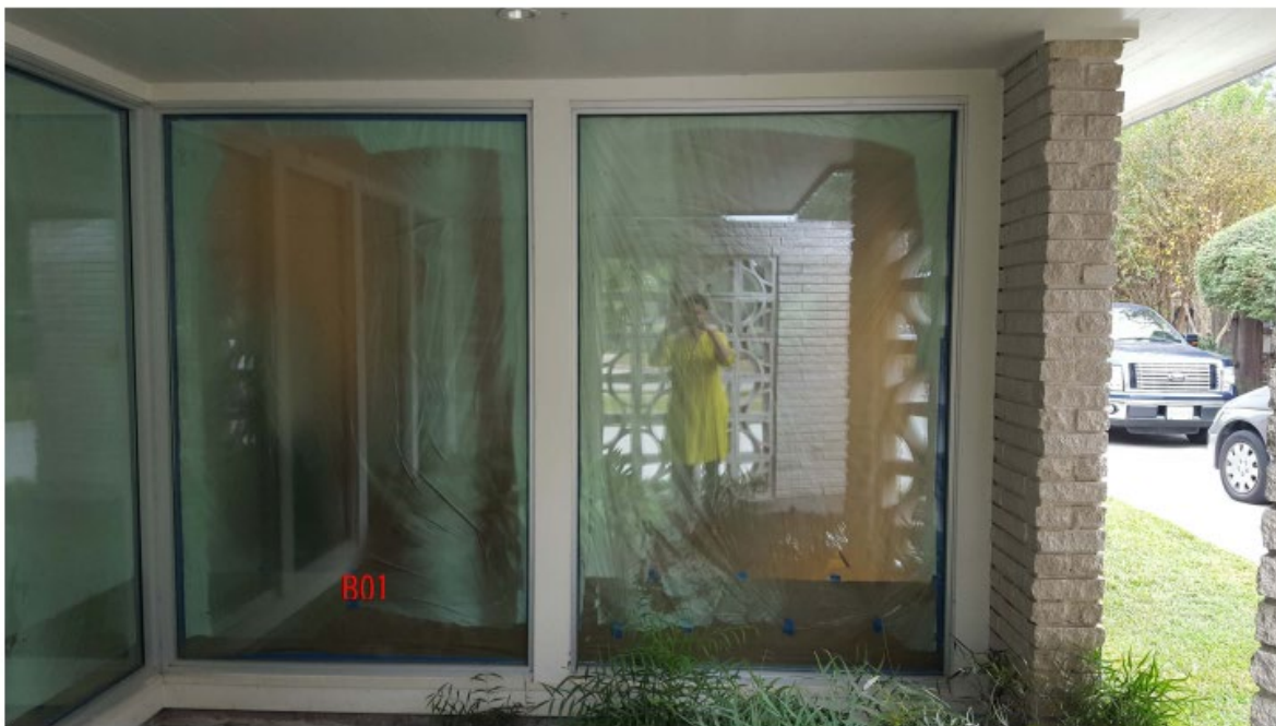
13 – West (side) elevation at side of house, showing window unit B01
