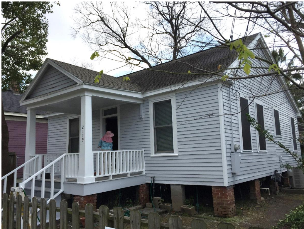
Figure 2 - Prior to current work-was residing previously with wood
