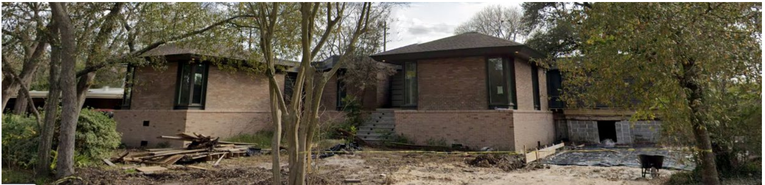
BEGINNING FOOTPRINT OF FORWARD GARAGE C.2021
