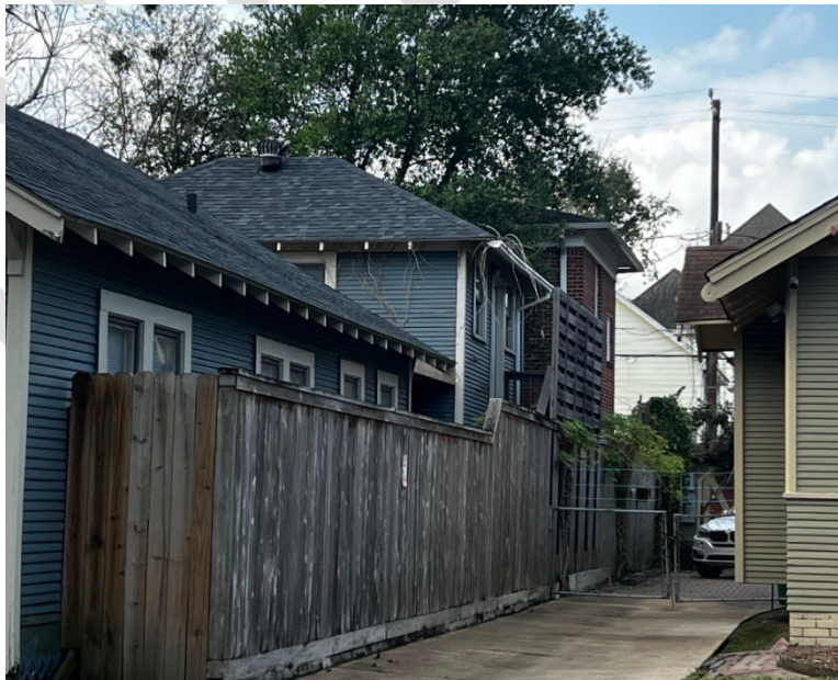
Figure 1- Side north elevation _ Privacy wall removed
