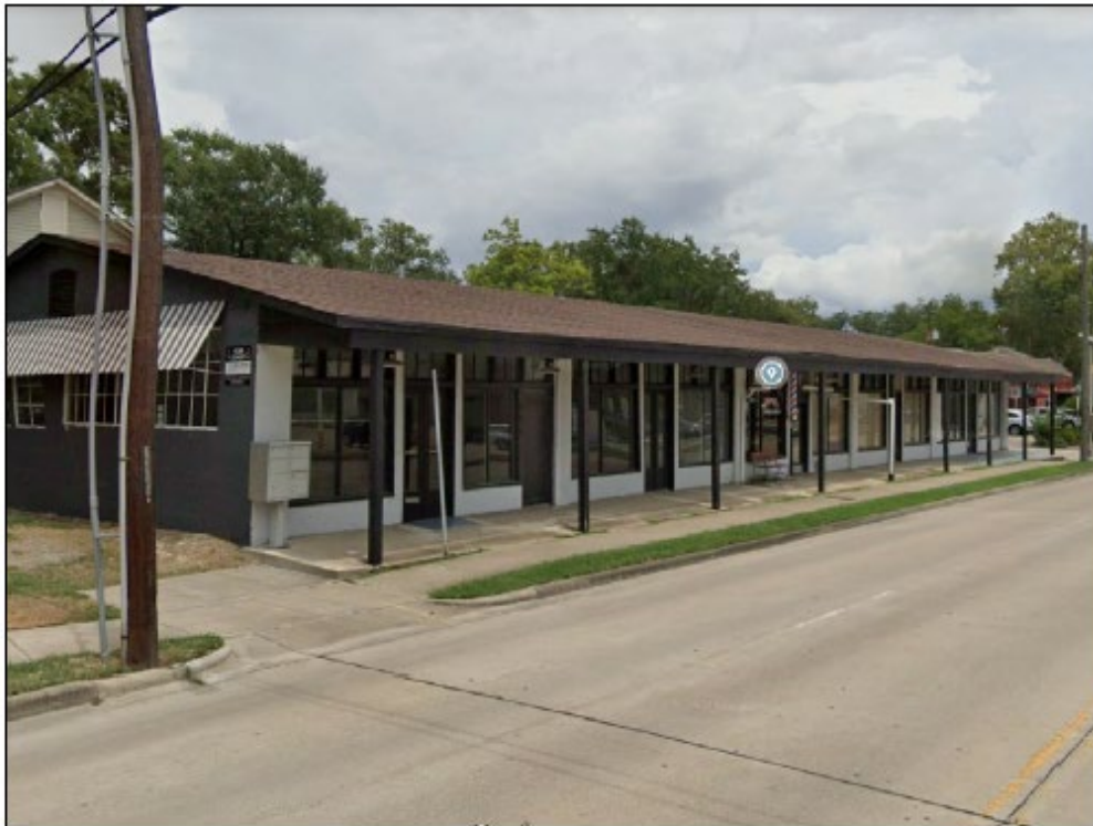
EXISTING 215 E. 11TH, CONTRIBUTING, ESTIMATED HEIGHT 13'-0", PAINTED EXPOSED CANOPY STRUCTURE SIMILAR TO PATIO
