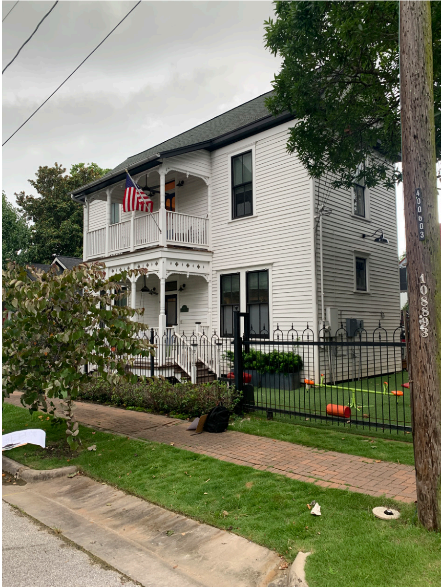
View from White Street of North Elevation
