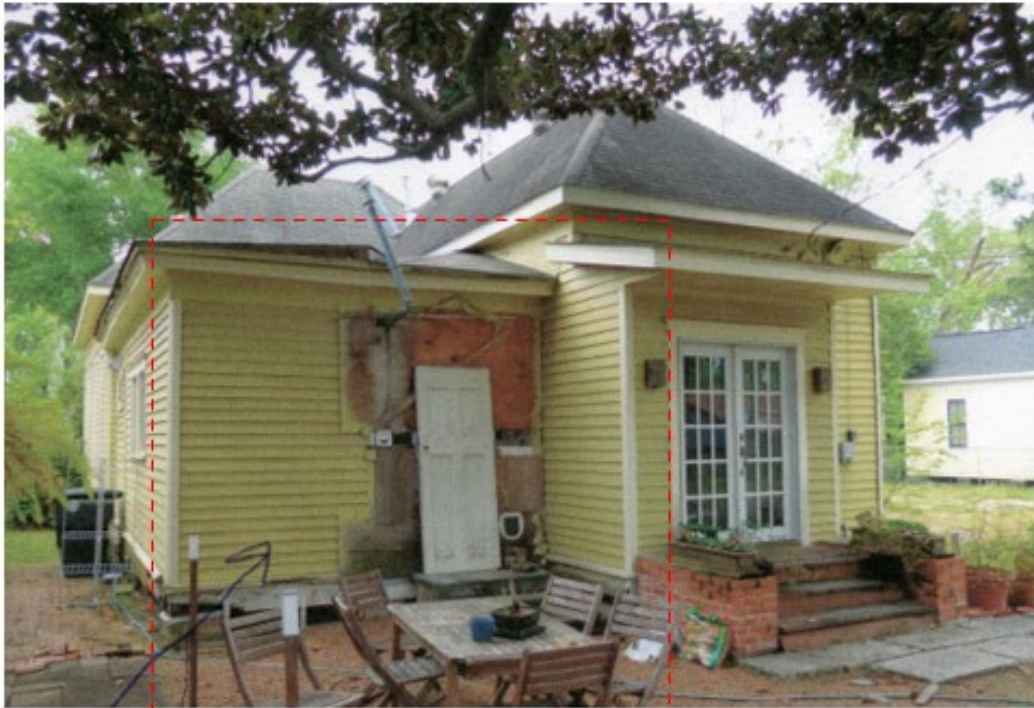
2013 Addition – Rear corner previously absorbed
