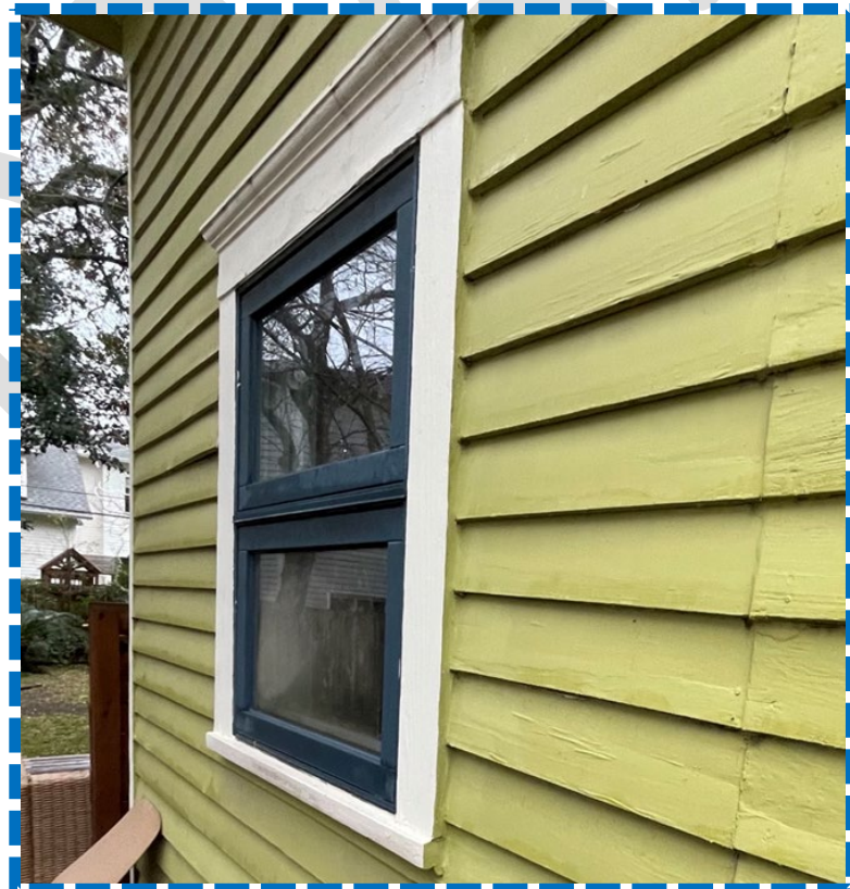
Non-original window/patched siding
