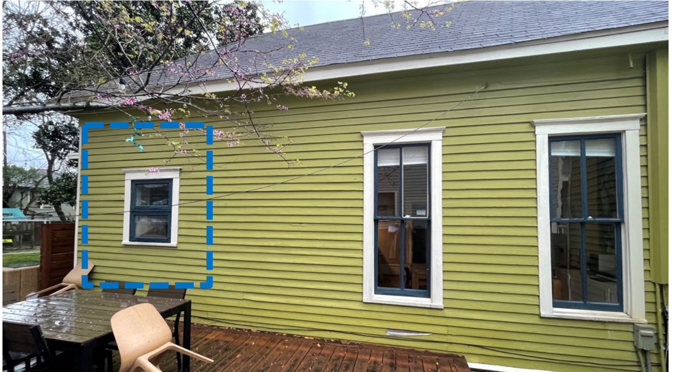
Non-original window/patched siding
