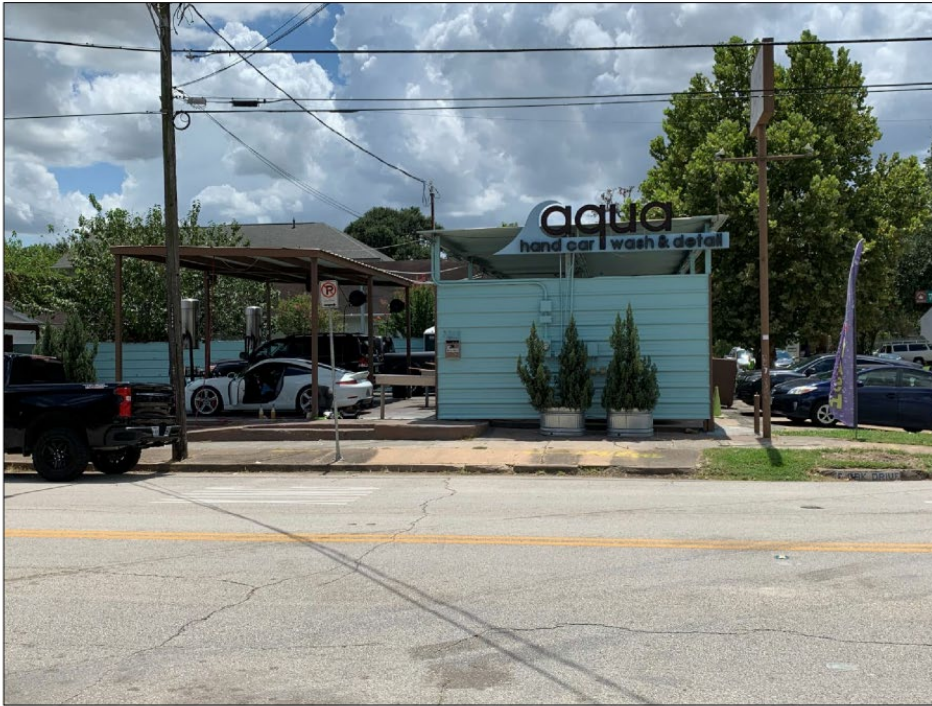
EXISTING CAR WASH BUILDING
