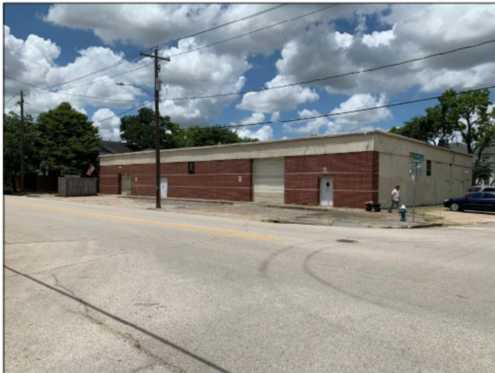
EXISTING 3400 WHITE OAK, CONTRIBUTING, ESTIMATED HEIGHT 18'-0", MIXED BRICK, CONTINUOUS EXTENDED PARAPET CAP
