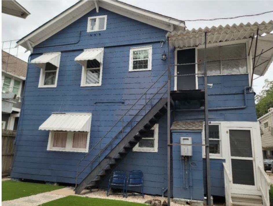
Back Side of Front Building
