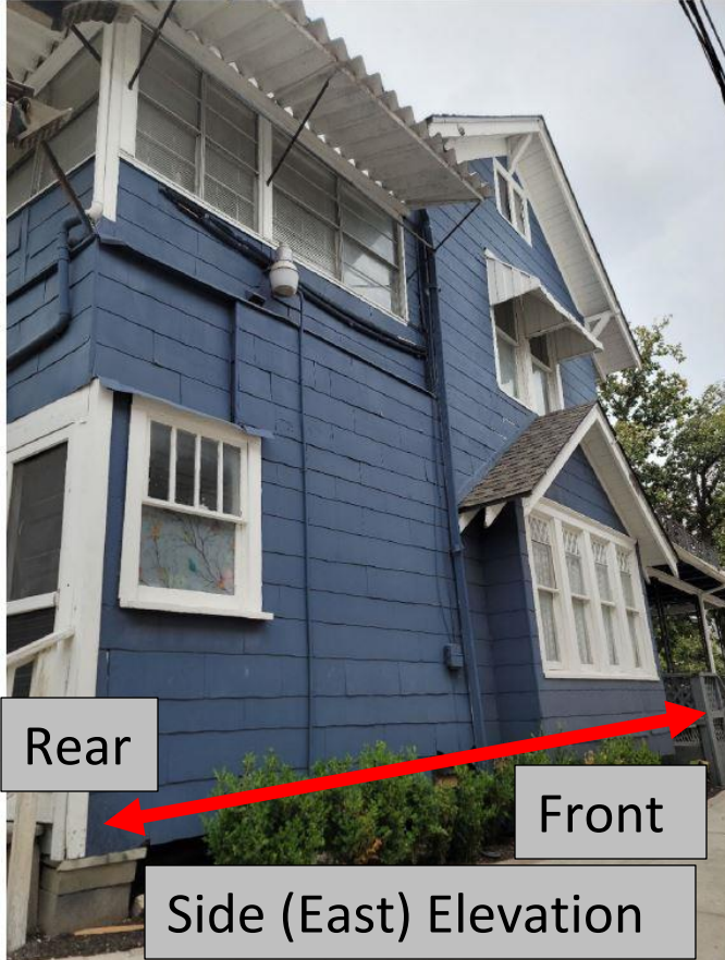
Eastern Side of Front Building
