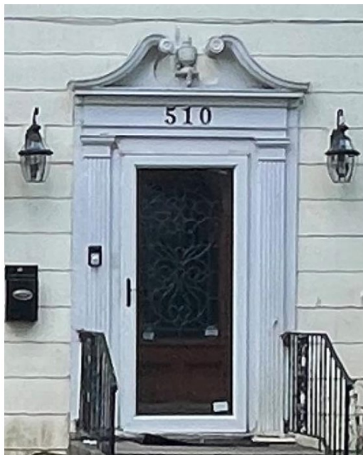
Figure 16 Main door, ornament and lamps to be removed.
