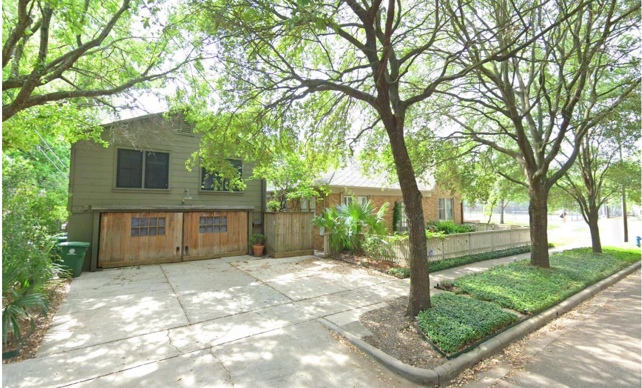
Figure 2 - Looking NW at garage apt and house
