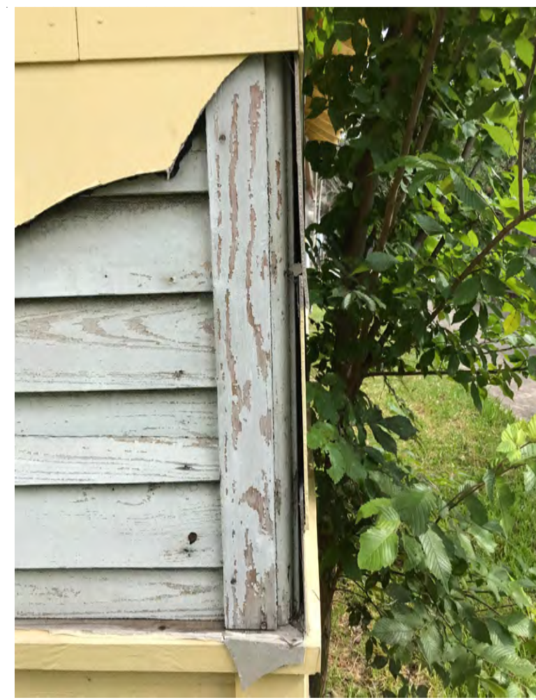
19 Existing Corner Boards NOT TO SCALE
