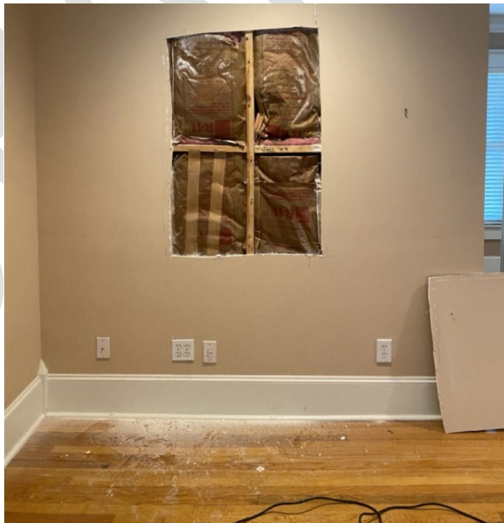
New Framing w/o Shiplap at Assumed Original Door Location
