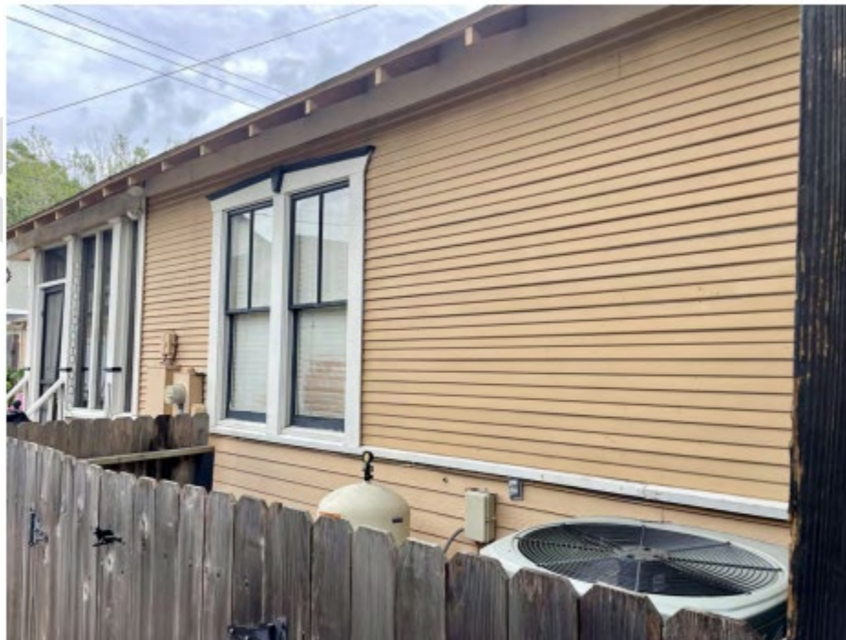
South Elevation - Behind Wood Fence
