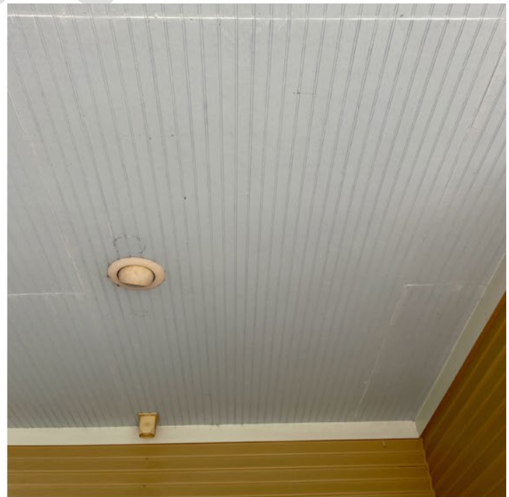
Front Porch Soffit (Non-contributing 4x8 bead board)
