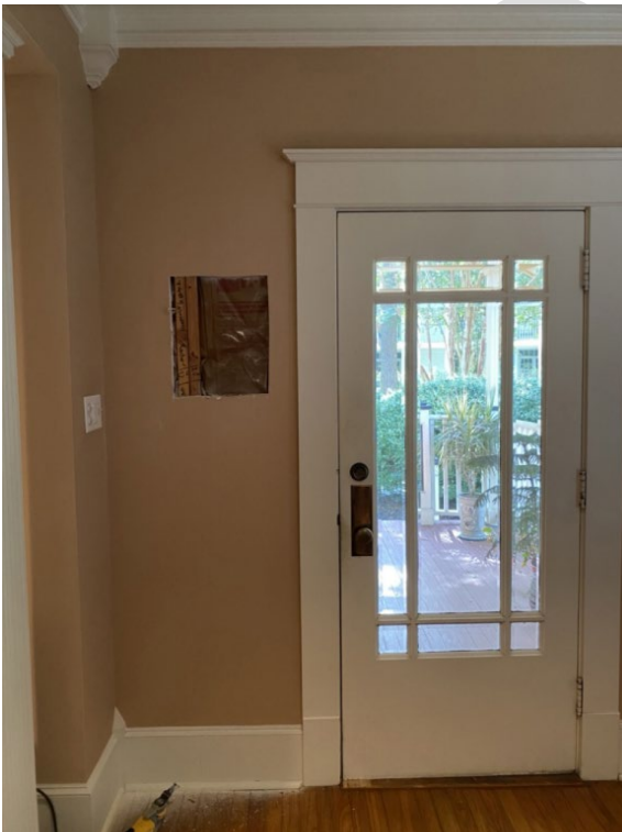
New Framing around Current Front Entry Door
