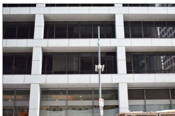
6. Tower, Lamar Street elevation, view N, photo taken from sidewalk across the street - imaged BRIGHTENED to increase visibility of mockup framing
