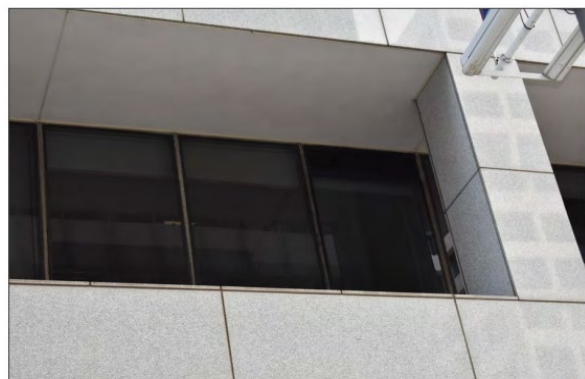
3. Tower, Lamar Street elevation, view N, close up photo taken from sidewalk directly in front of building
