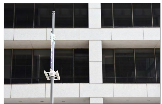
12. Tower, Lamar Street elevation, view N, close up photo taken later in the day from sidewalk across the street - imaged BRIGHTENED to increase visibility of mockup framing
