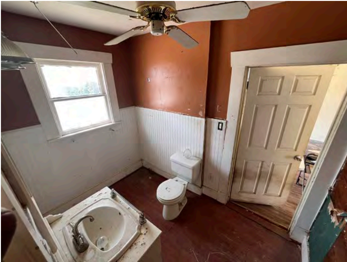
Figure 14 - Interior Photo from Applicant Provided Report, Appendix L
