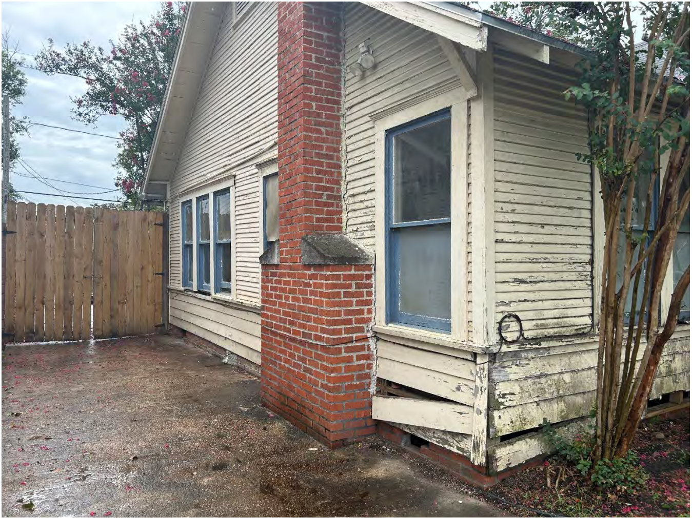
Figure 7 - Staff Photo East Elevation Corner
