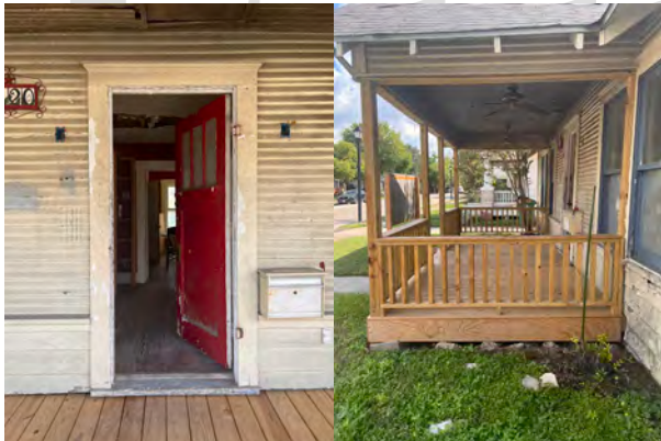
Attic access hatch from the front porch.
