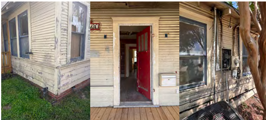
View of subject property exterior siding.
