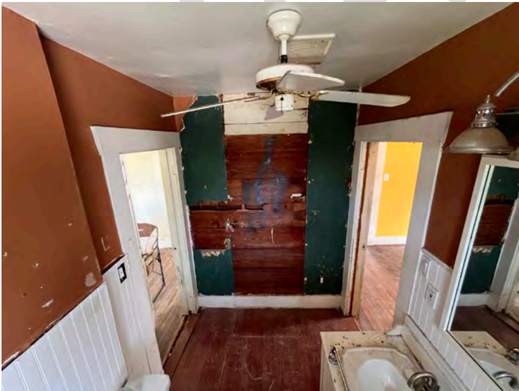
Figure 13 - Interior Photo from Applicant Provided Report, Appendix L
