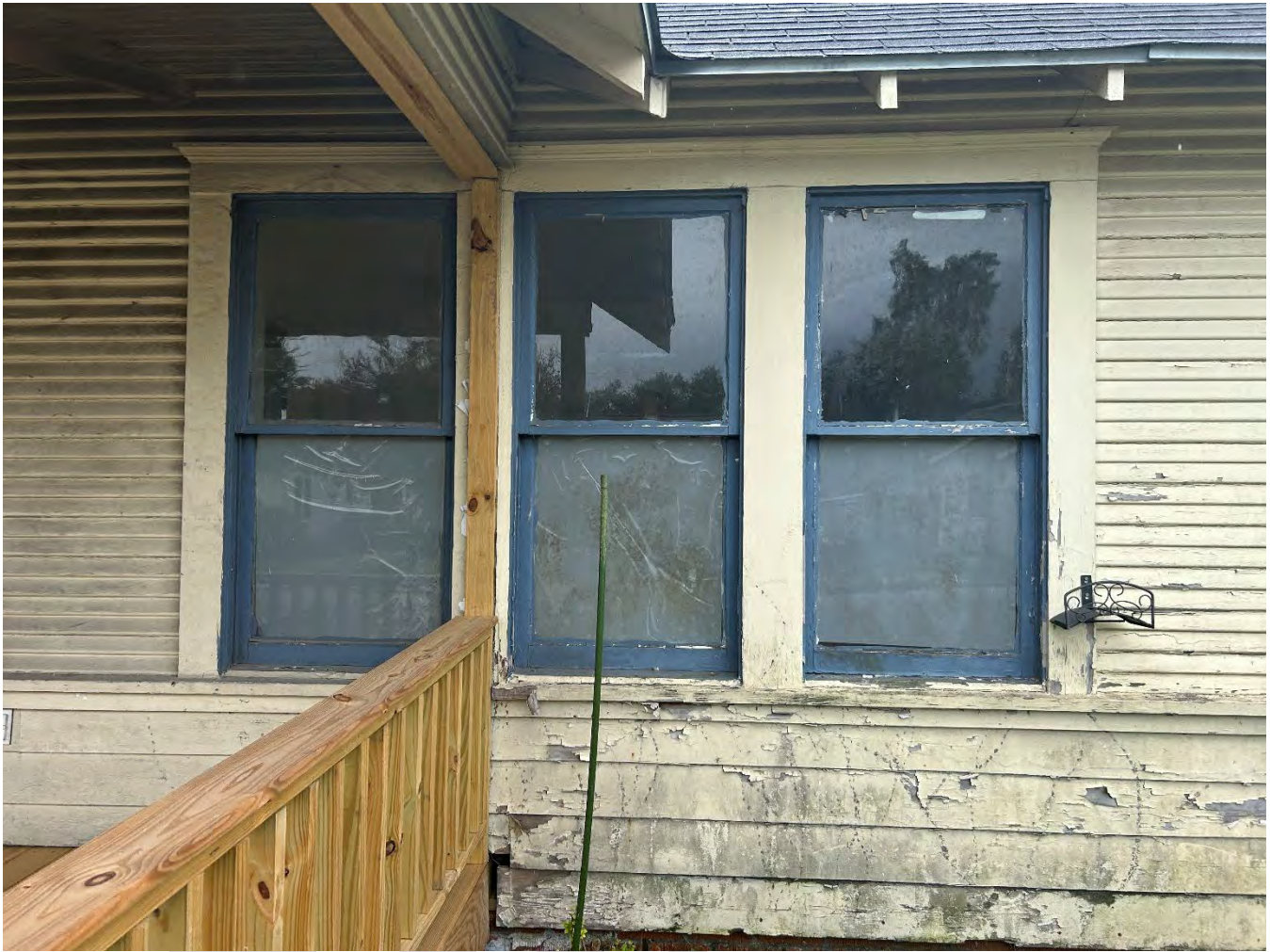
Figure 4 - Staff Photo Front Right of House
