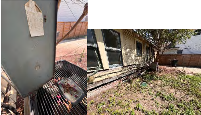
HVAC system for the subject property
