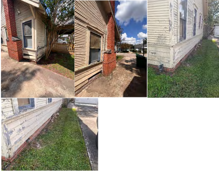
Foundation area for the subject property.
