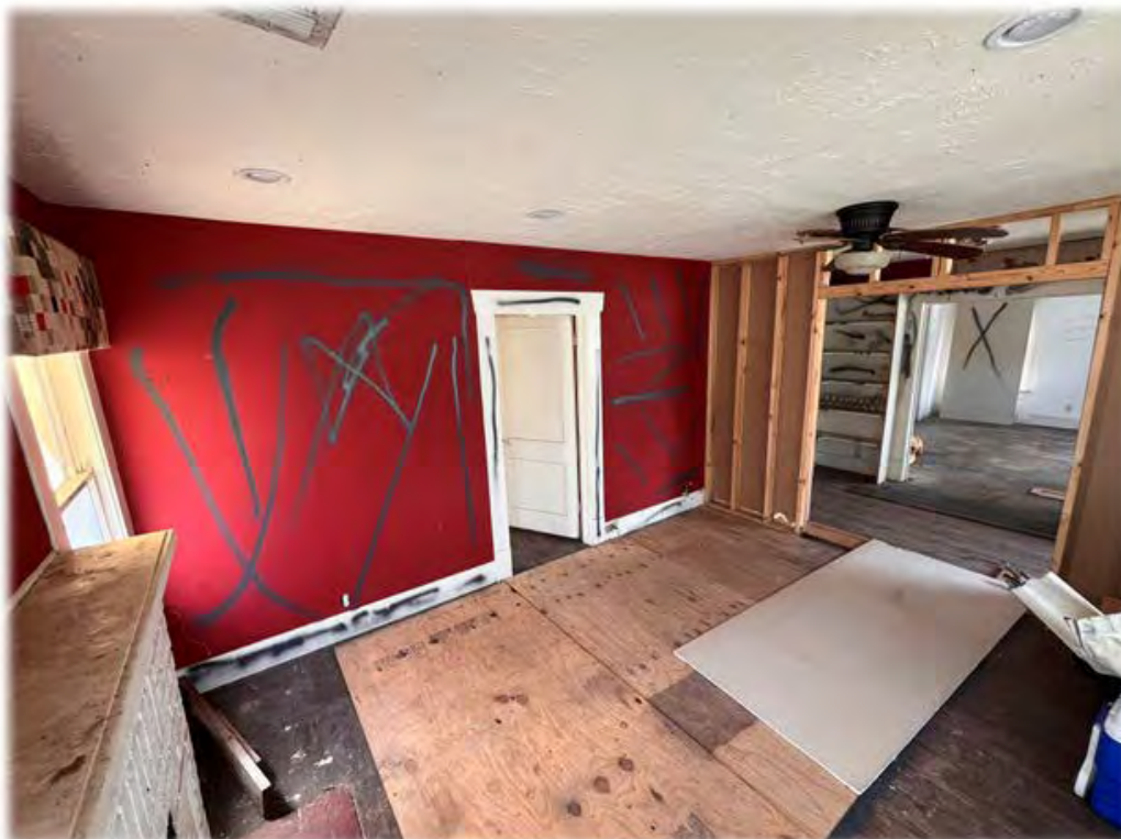
Figure 11- Interior Photo from Applicant Provided Report, Appendix L
