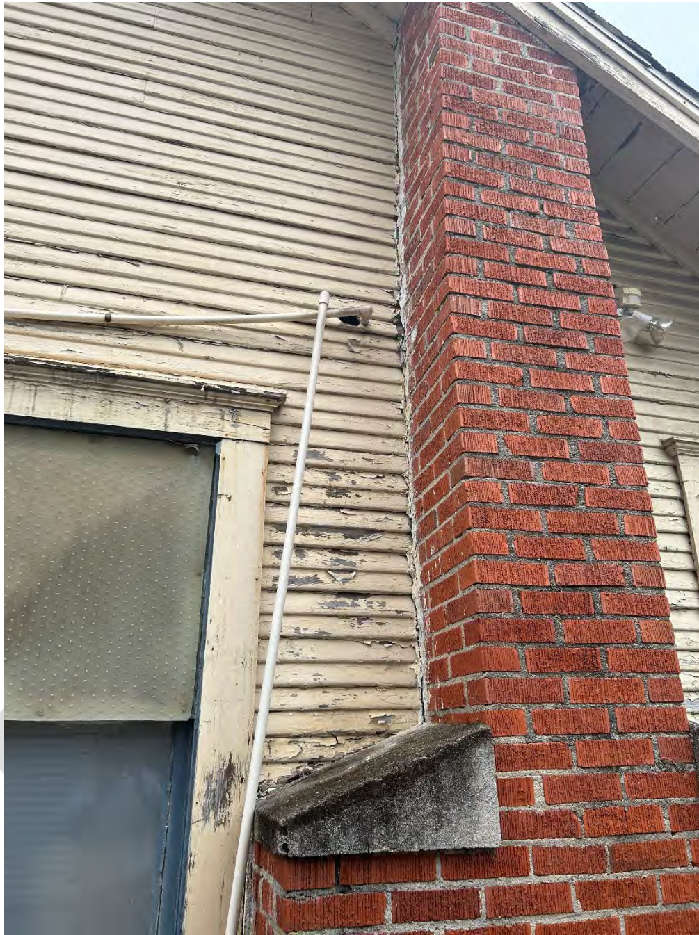
Figure 8- Staff Photo East Elevation Detail
