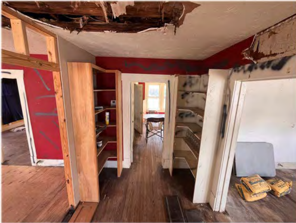
Figure 10 - Interior Photo from Applicant Provided Report, Appendix L
