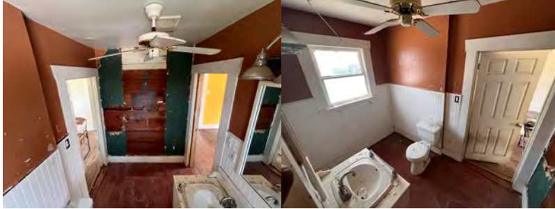
Subject property bathroom.
