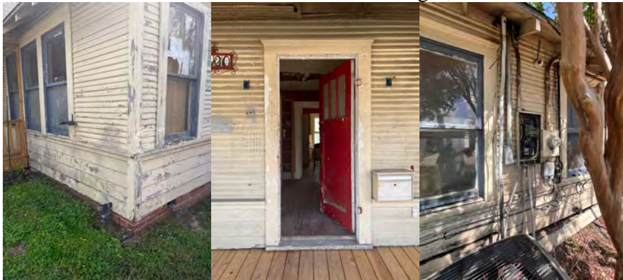
View of subject property exterior siding.
