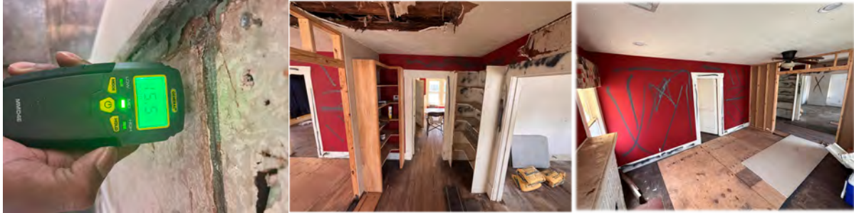
Subject property interior walls and conditions.
