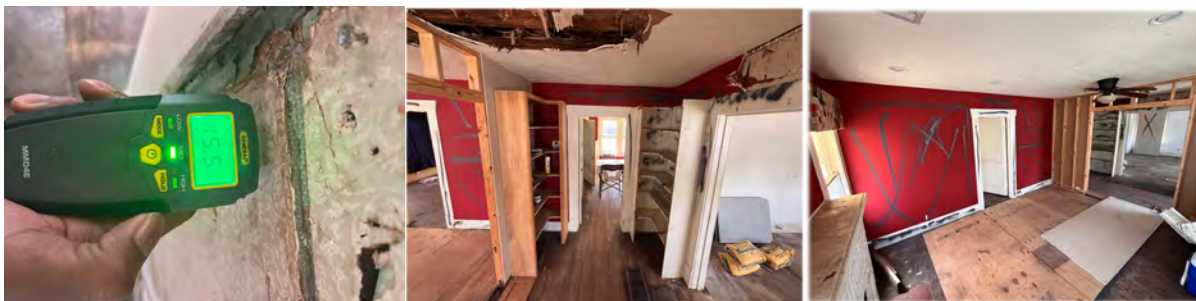
Subject property interior walls and conditions.
