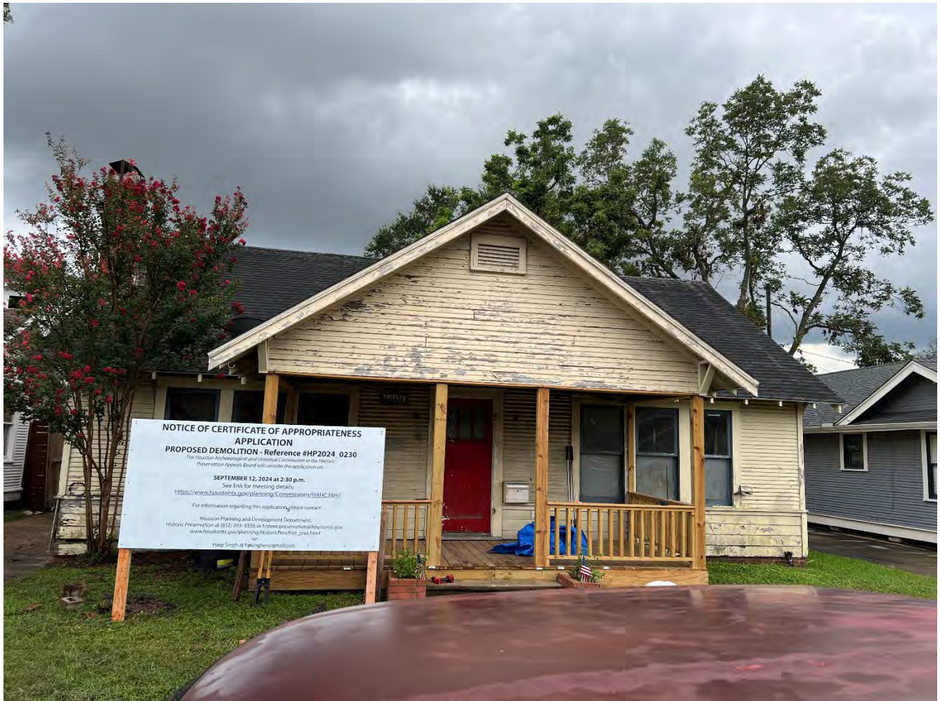
Figure 2 - Photo from Applicant with Required COA Demolition Notice
