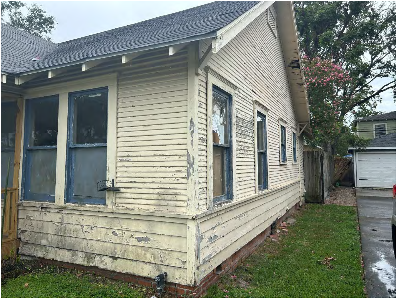
Figure 5 - Staff Photo West Elevation Corner
