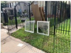
Removed Windows 6a
