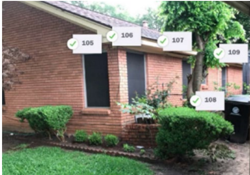
FRONT – RIGHT SIDE (EAST & NORTH ELEVATIONS)
