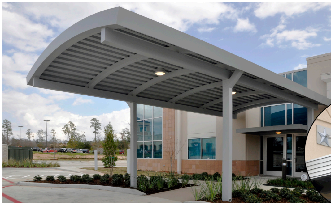
Creekside Surgery Center, Browne McGregor Architects
