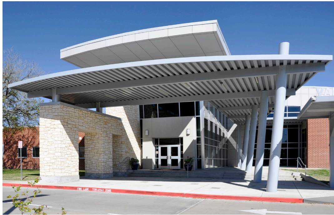
Valley Oaks ES, PBK Architects
