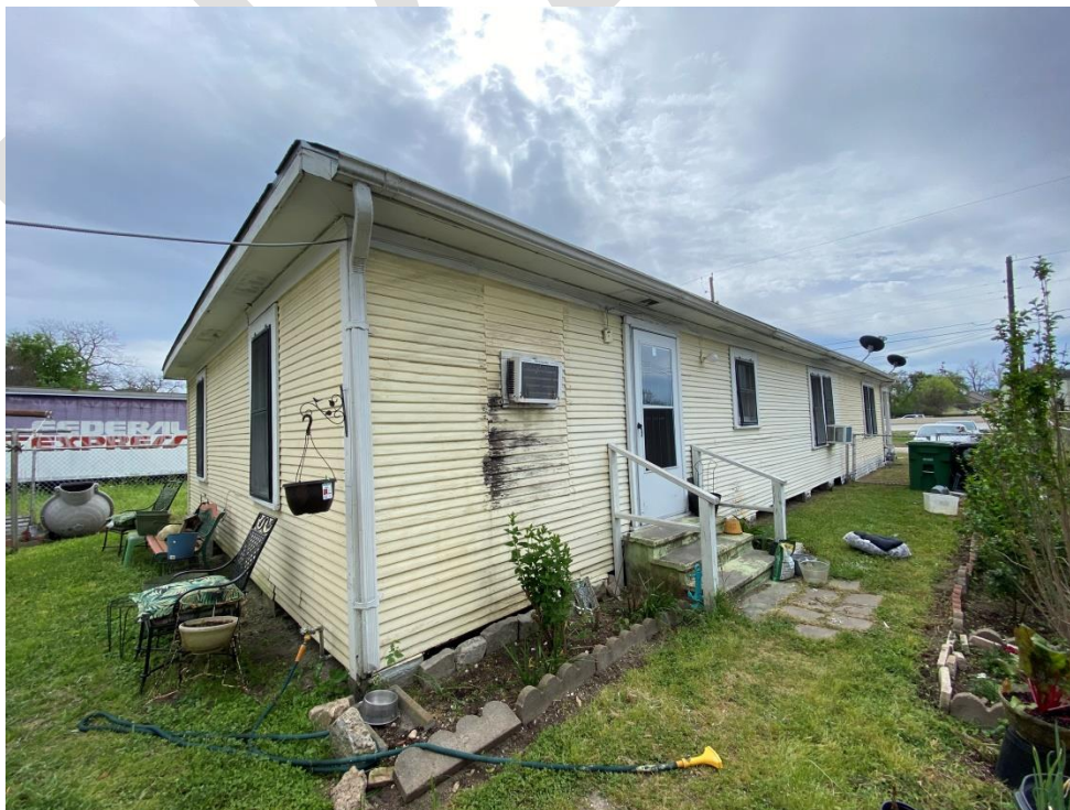
Photograph 2. View facing southeast.
