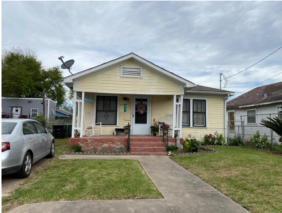
Photograph 1. View facing north.
