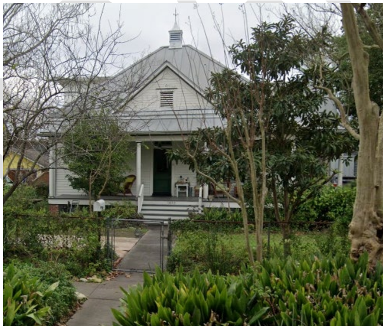
Figure 2- 1842 Cortlandt next door neighbor
