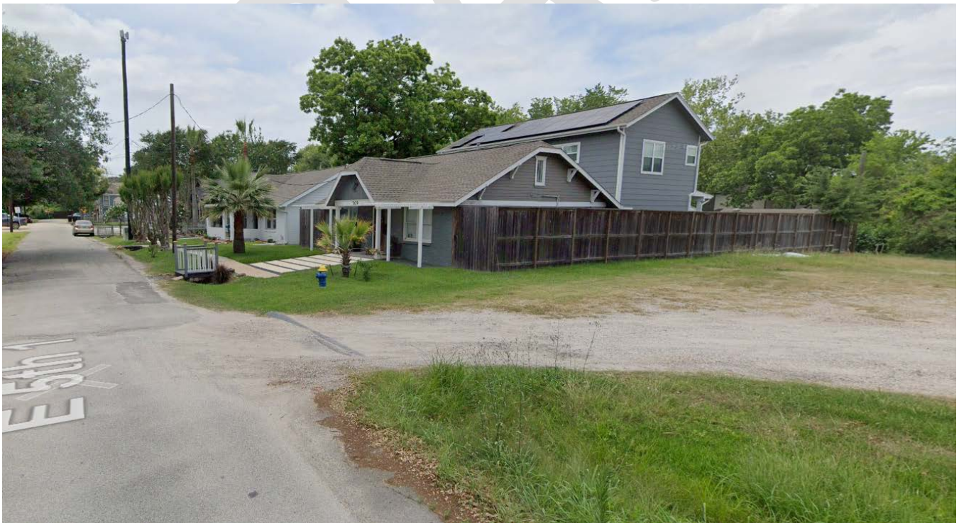
Figure 2_ View from E 5th 1/2 St
