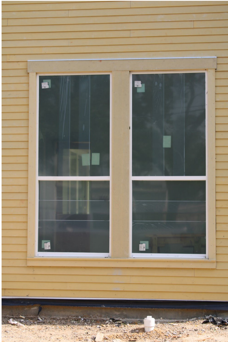
FRONT ELEVATION WINDOWS, CONTINUED
