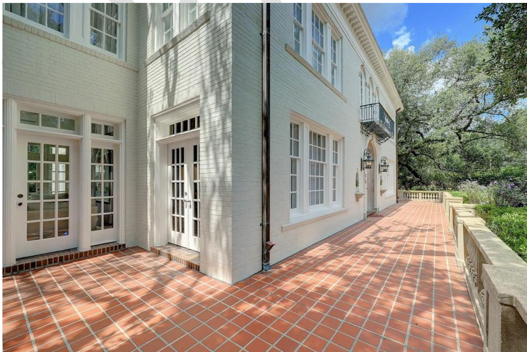
EAST (FRONT) ELEVATION – OBLIQUE FRONT PATIO – LOOKING NORTH
