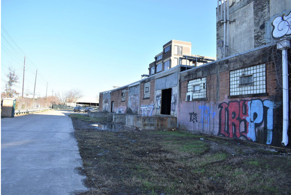
Photo 3 Swift & Co. Packing Plant; North elevation; view east
