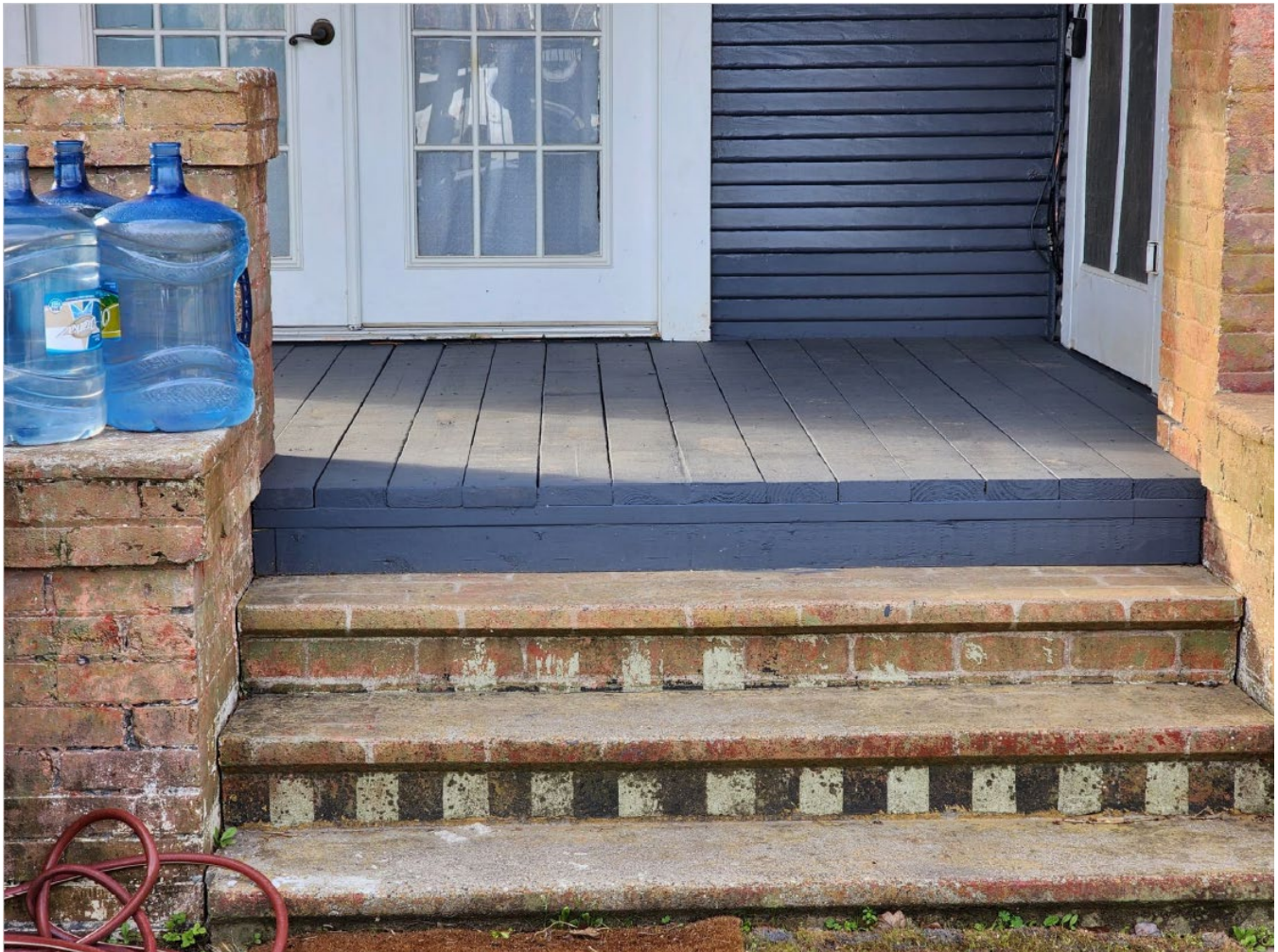
Figure 4 - Close up of new decking
