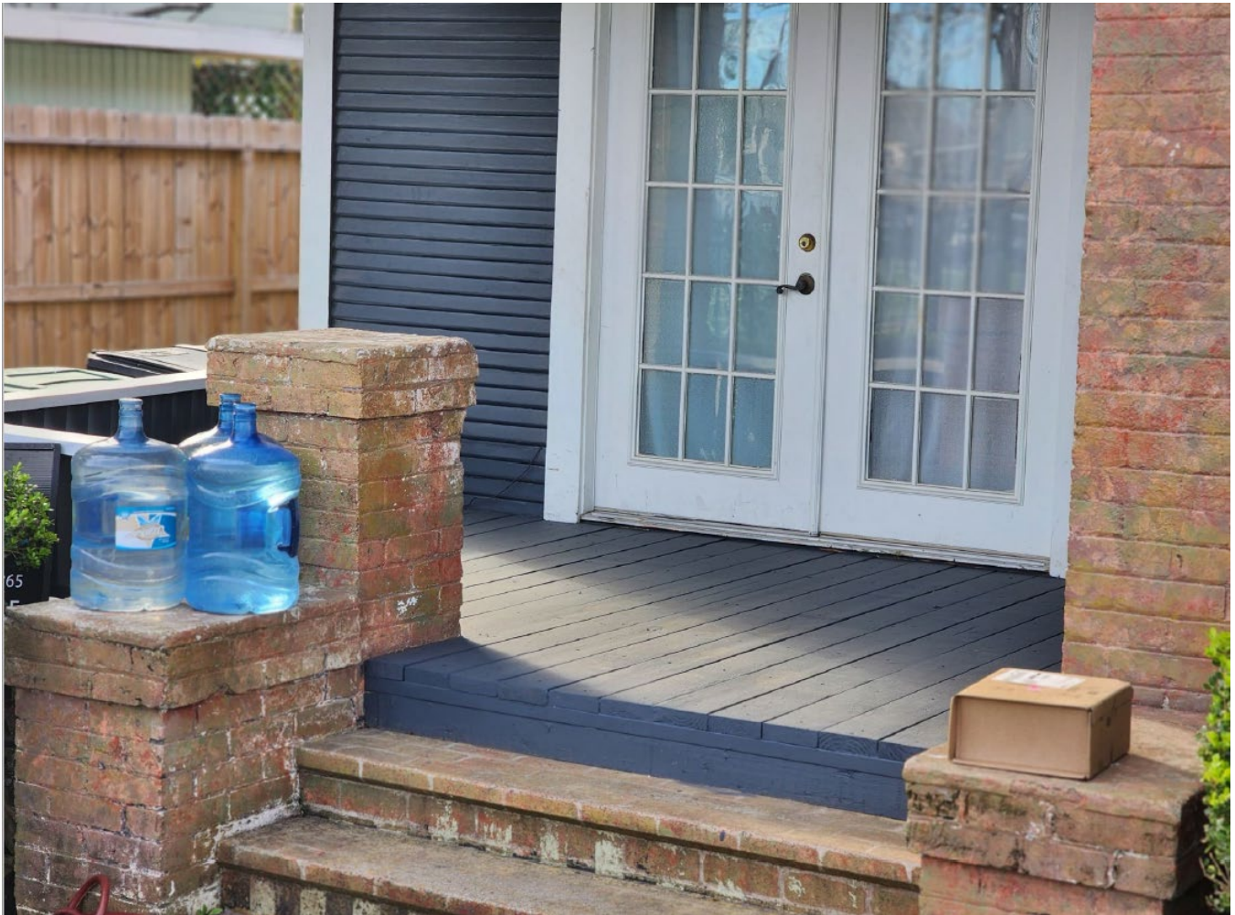
Figure 5 - Additional View Close Up of Decking
