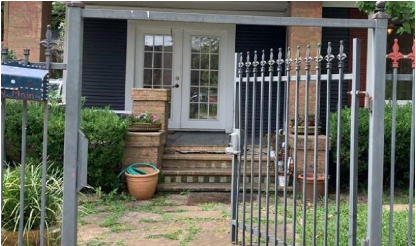
Figure 2 - View of Porch Floor Prior to Alteration
