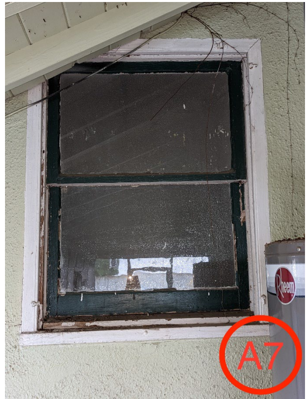
Figure 15 - Window on Rear Porch
