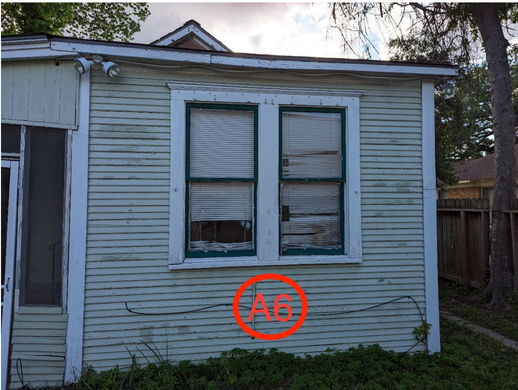
Figure 13 - Non-Original Rear Addition
