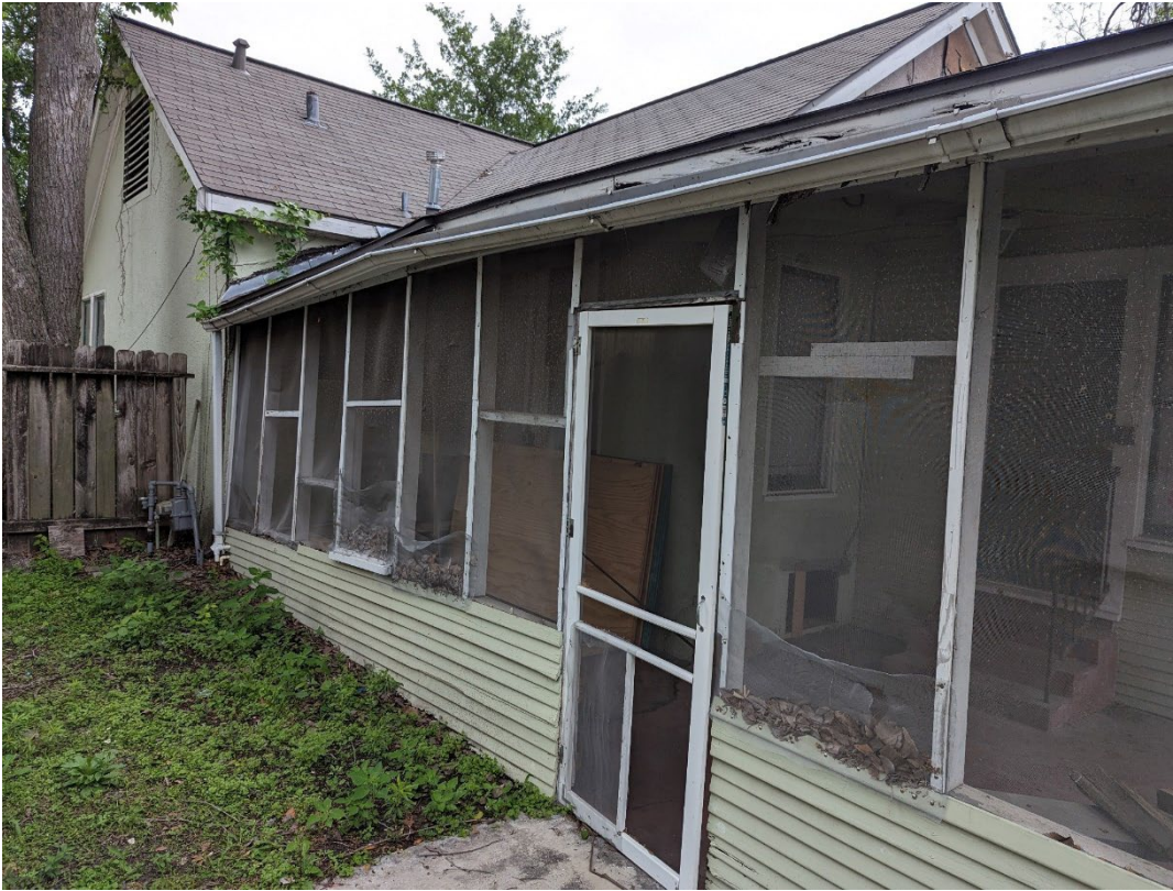
Figure 12 - Covered Porch Non-Original
